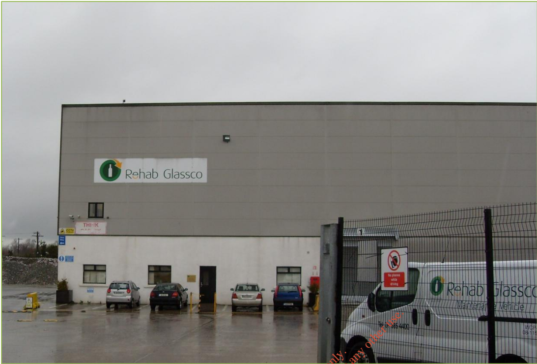
Photograph 2.3: Main Process Building (including offices)
