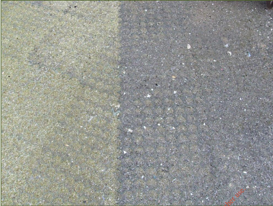
Photograph 2.45: Plastic Ground Matting System at Wayleave
