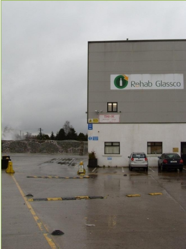
Photograph 2.37: Site roads and concrete hardstanding
