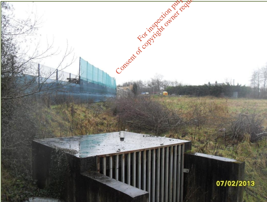
Photograph 2.46: Culvert located in field to north-west of Rehab Glassco site
