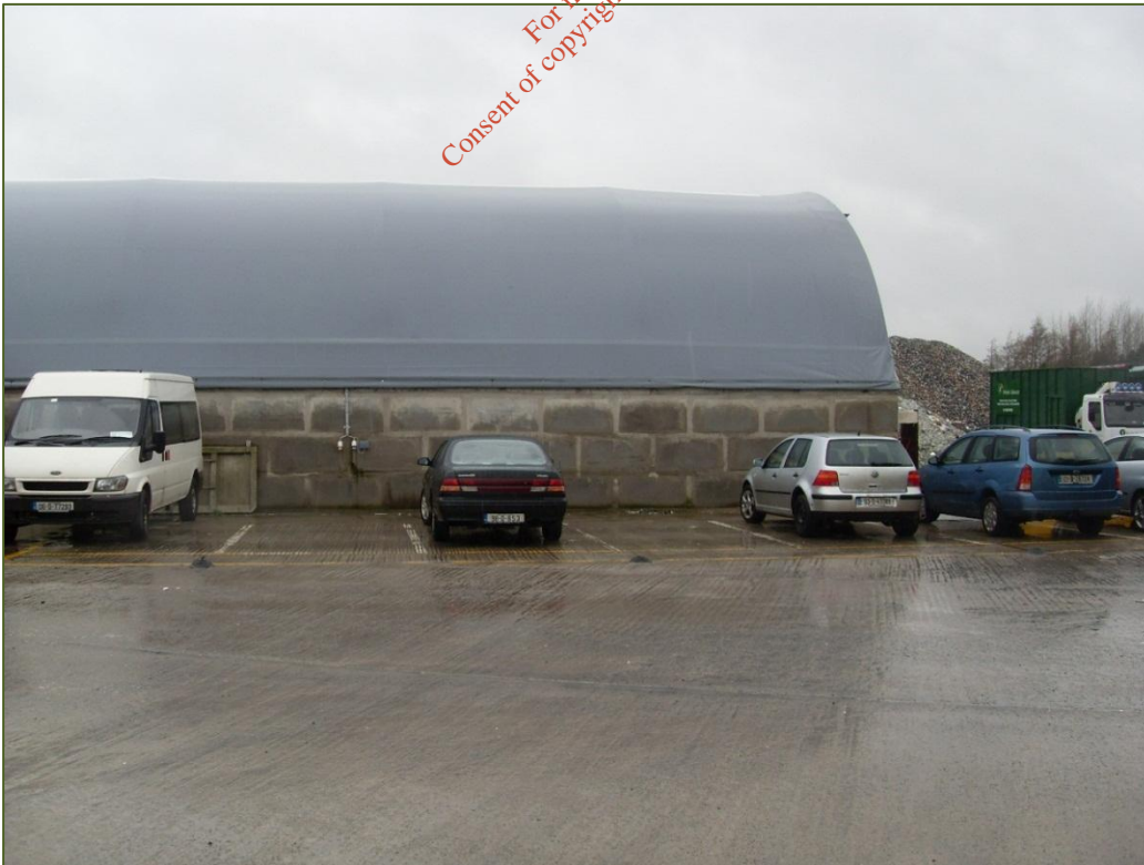
Photograph 2.38: Designated parking area
