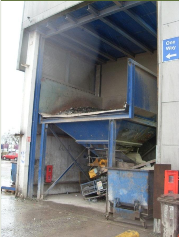
Photograph 2.9: Main Process - Loading Hopper into Main Process
