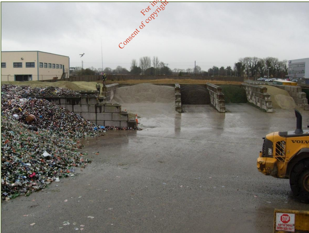
Photograph 2.26: Input and Output Storage Bays, Concrete Hardstanding
