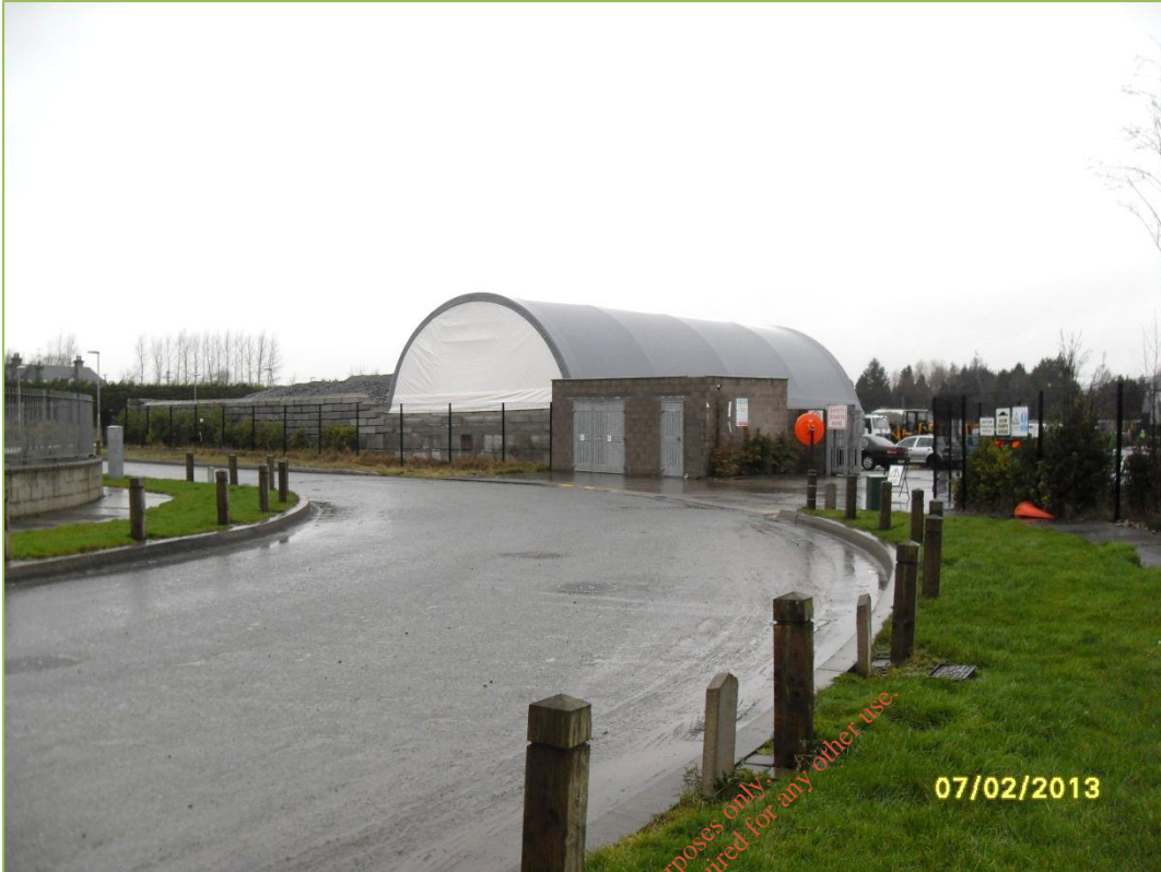
Photograph 2.1: Access road, Osberstown Industrial Park
