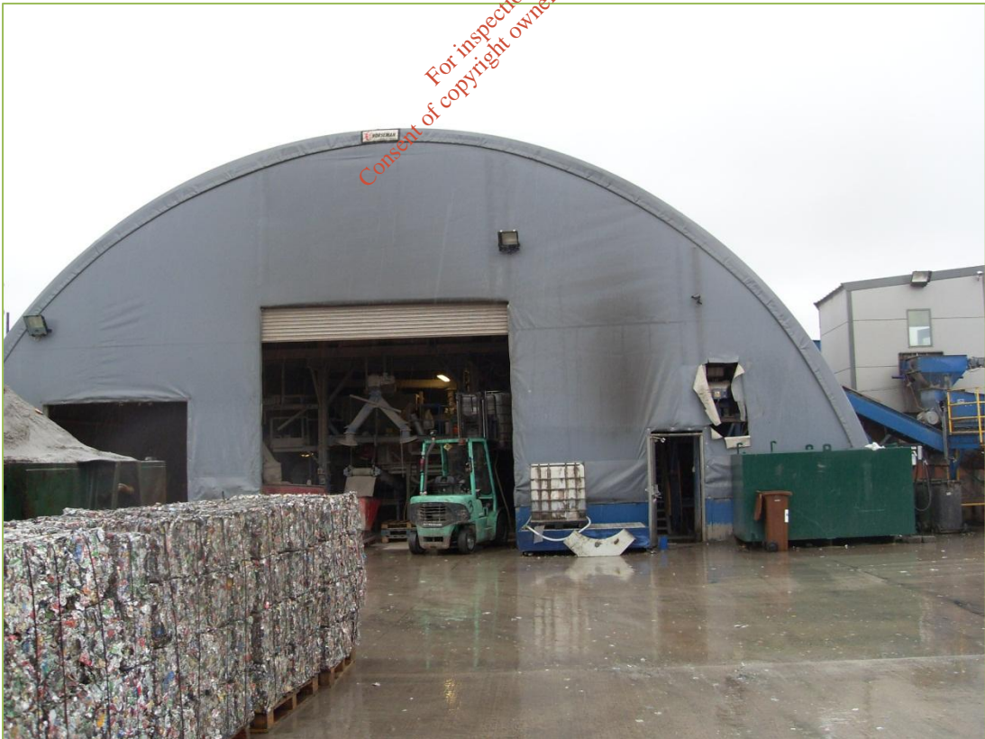
Photograph 2.4: Drying Plant Building
