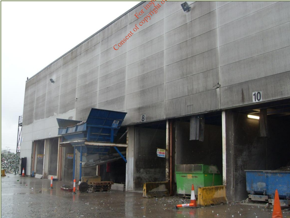
Photograph 2.20: Main Process Building - Output Bays
