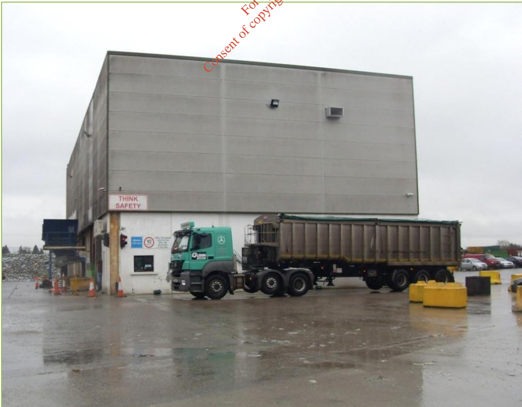
Photograph 2.6: Main Process Building - Weighbridge position and weighbridge operator's window
