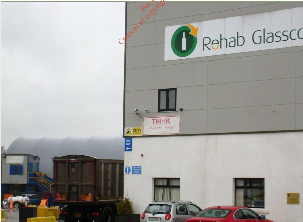
Photograph 2.40: CCTV camera positions on Main Process Building
