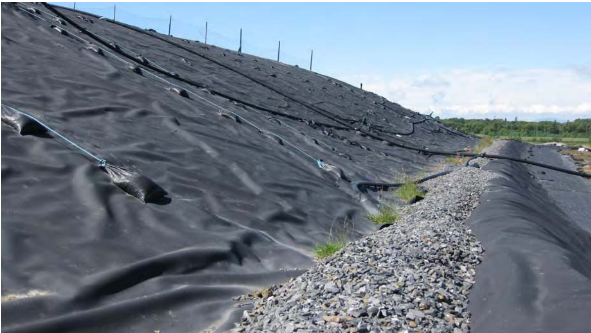
Photograph 4 : Temporary Cap Phase 5 Cell 3
