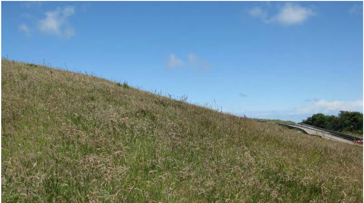
Photograph 2: Capped Area Phase 4
