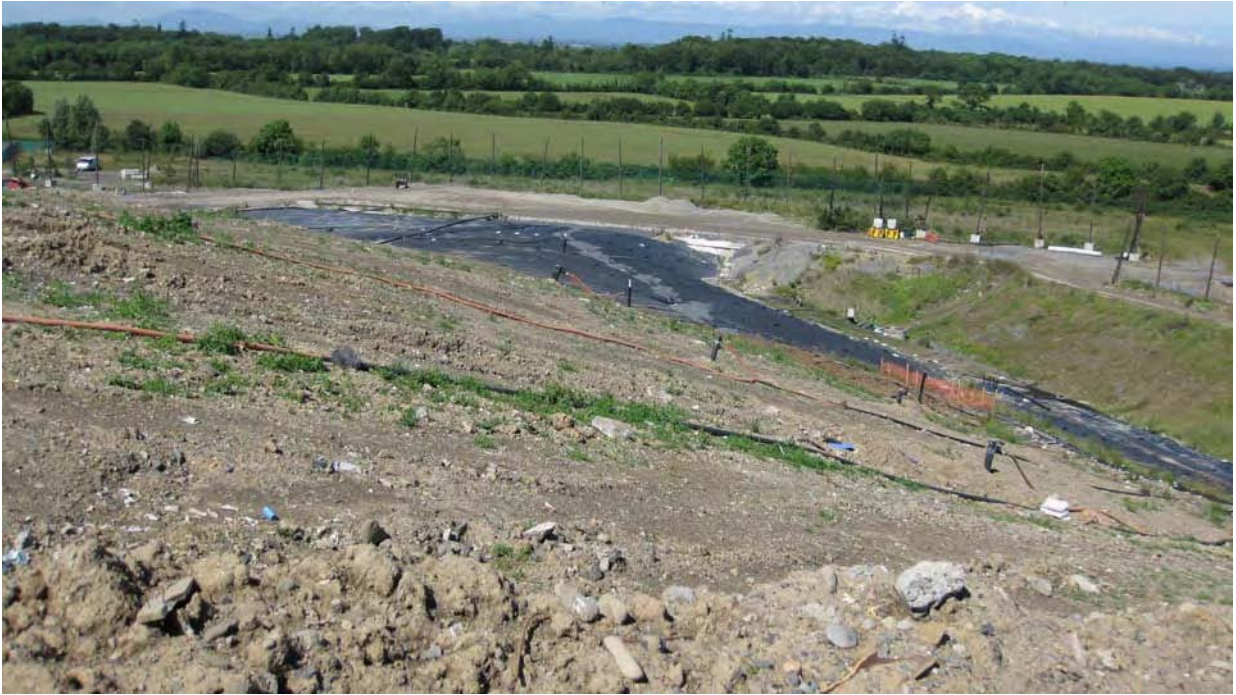
Photograph 5: Existing Waste Slope Cell 2B
