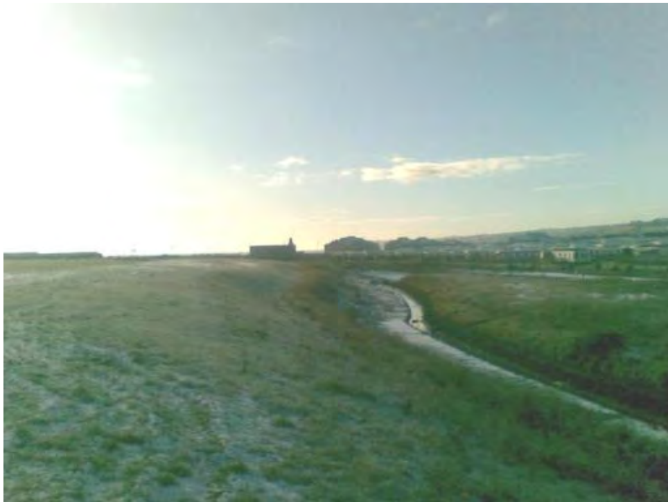
Slope Section 1 looking South
