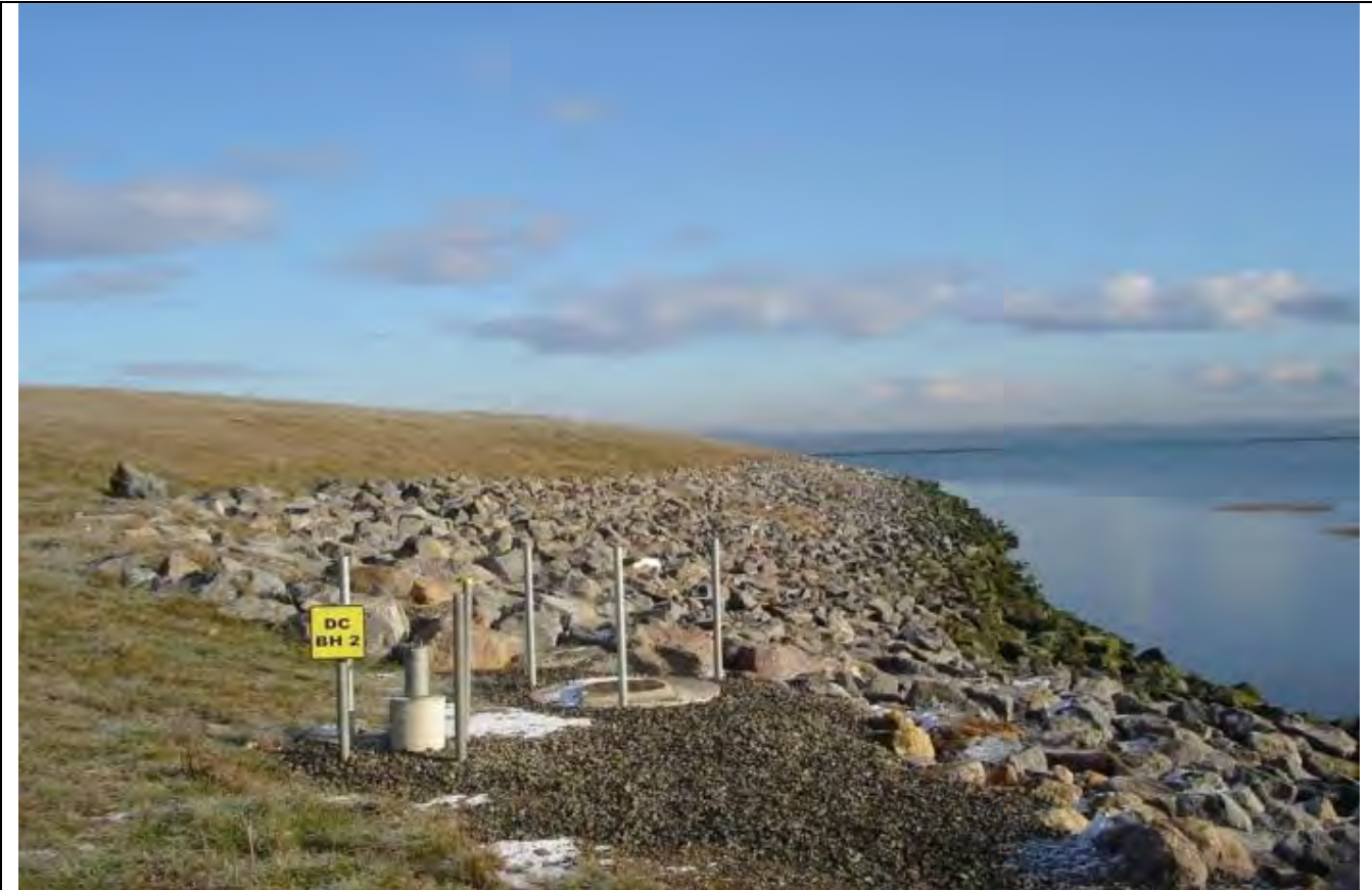
Slope Section 6 showing Rock Armour
