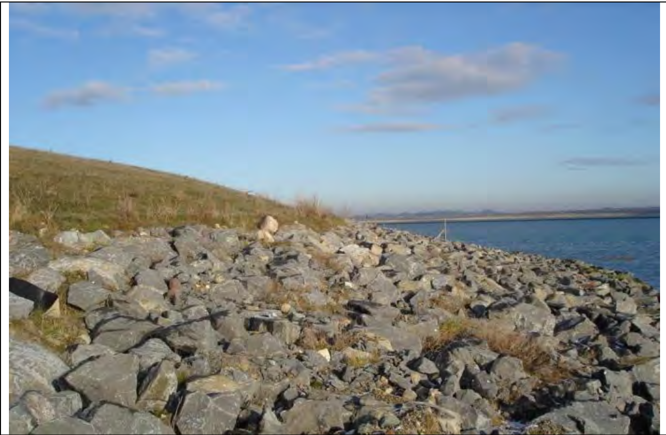
Slope Section 5 with Rock Armour.
