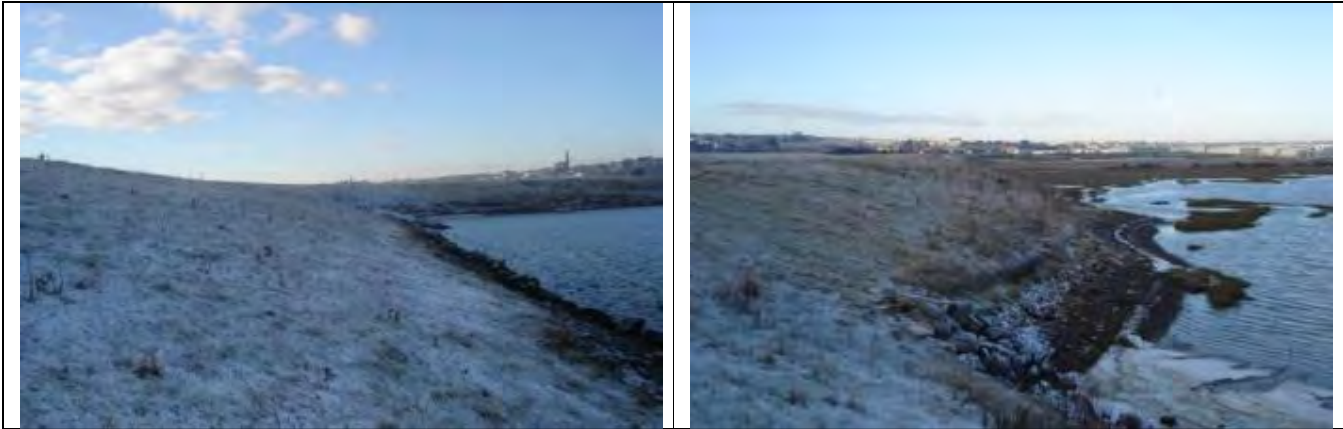
Slope Section 3 showing the Surface Water drainage outfall.
