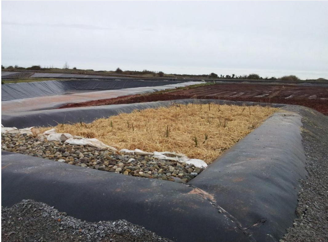
Plate 1. Wetland cell constructed on BRDA. Vegetation is currently in the establishment phase.
