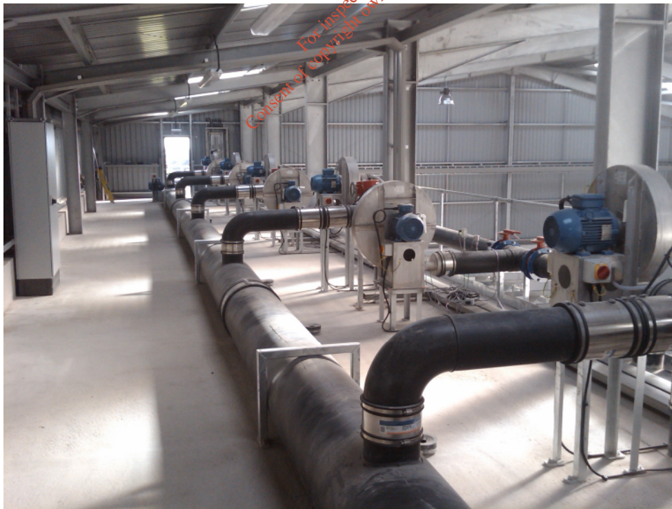
Fig. 16. The blower modules in the gallery of the Deepmoor tunnel composting facility in Devon.
