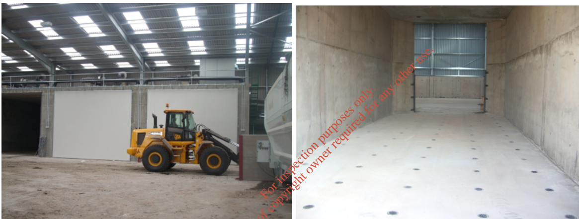
Fig. 15. Exterior of the composting biocells illustrating the sliding doors (left) and the proprietary C:N in-pavement aeration system (right).
