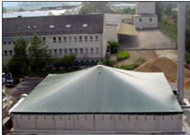
Figure 1: Typical enclosed Biofilter with Stack
