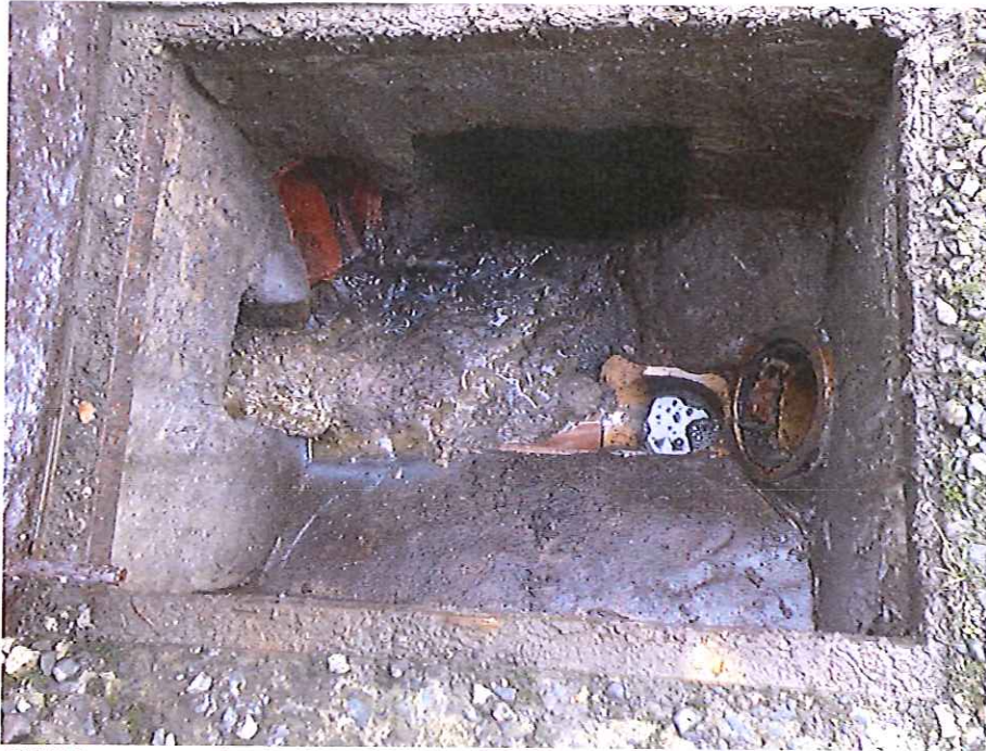
CSO1 prior to decommissioning of CSO works, Sept. 2011.
