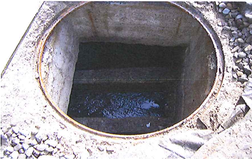
CSO3 , prior to decommissioning, March. 2008.
