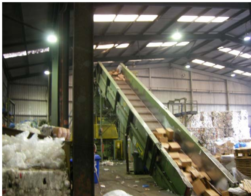
Figure 2.4: Baling Plant area
