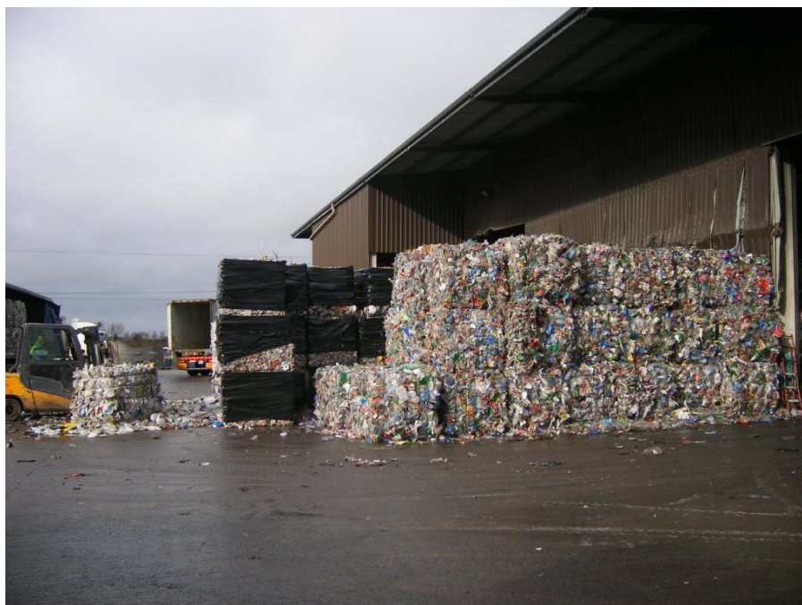
Figure 2.8: Canopy area over bale storage
