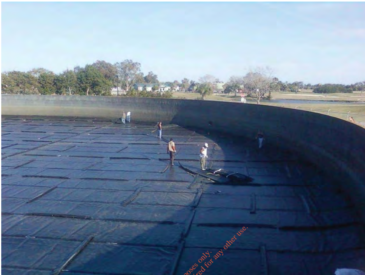
Figure 4.2 Example of covers for SBRs (source: Lemna Technologies Inc.)
