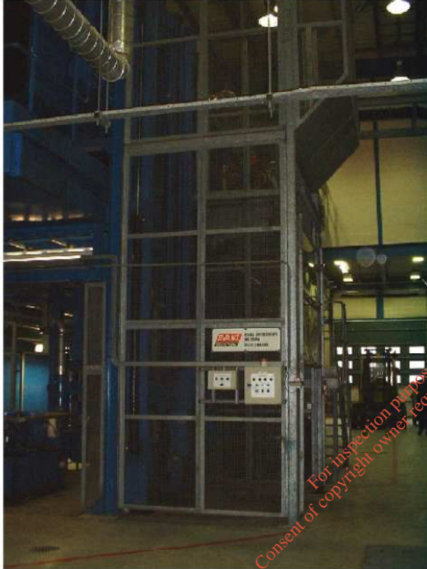
Lift to Direct Feed to Hopper
