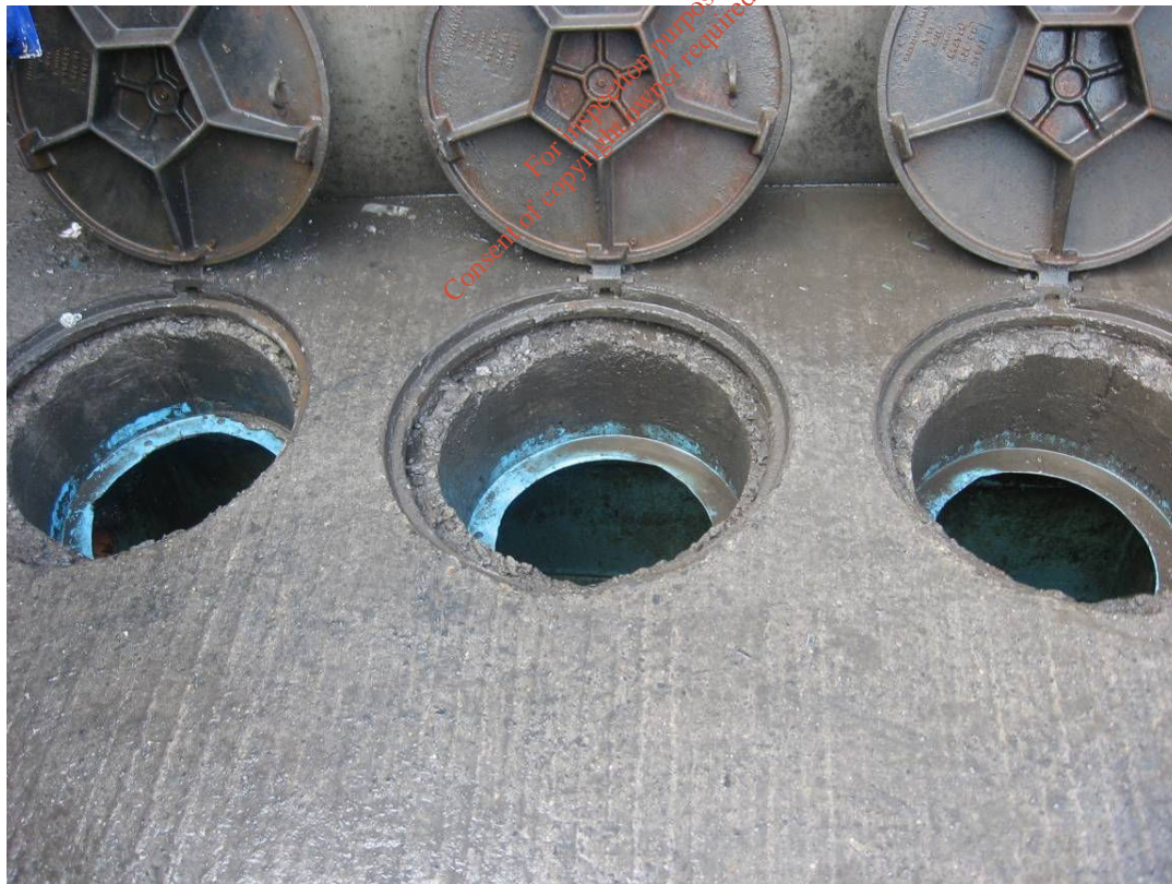
Plate 2.6.5-1: view of the manhole covers open at the CX interceptor unit
