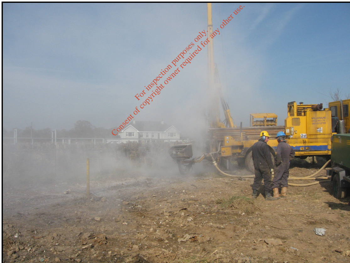
Photo showing Installation of GW2
