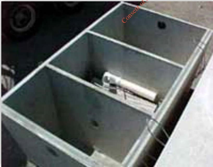
TRIPLE CHAMBER OIL INTERCEPTOR
