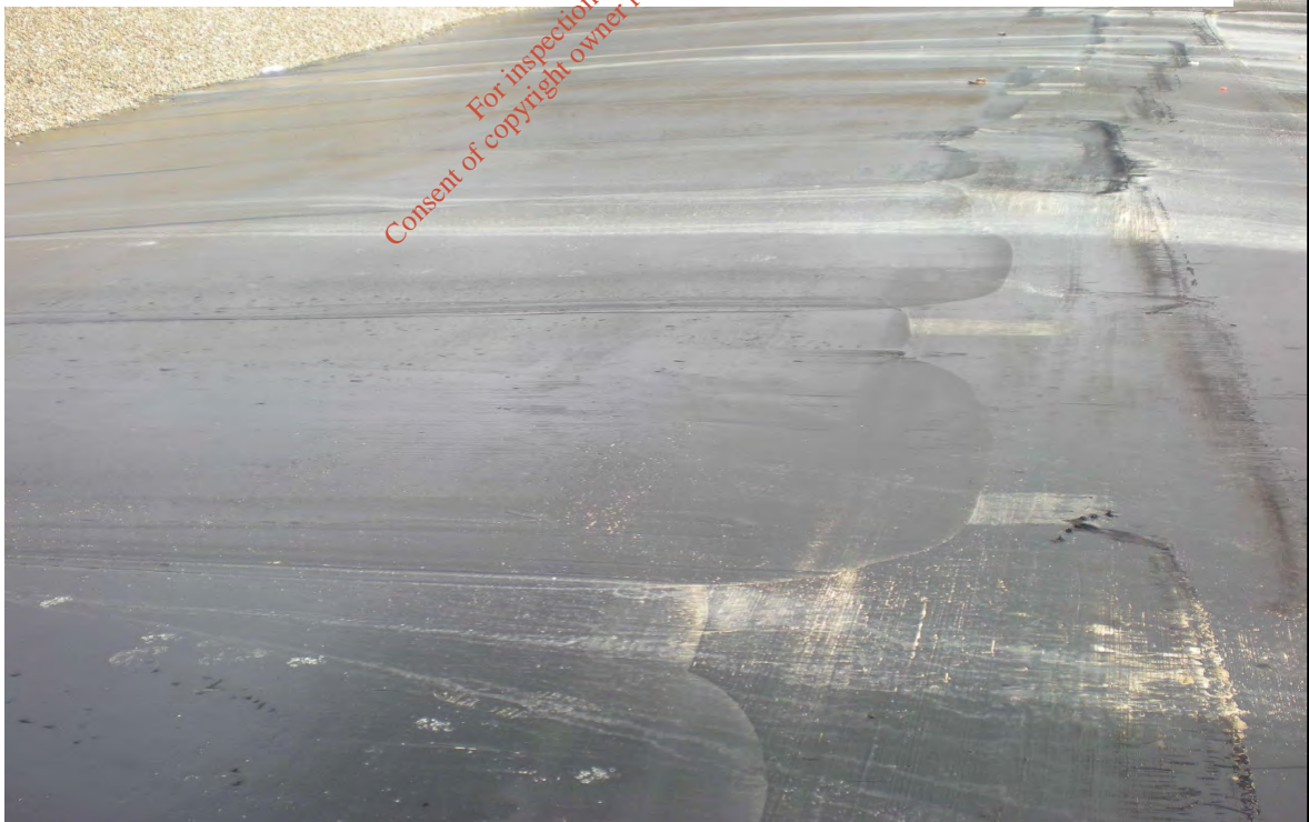
Photo 1 Lining of landfill cells with DAC at a UK Landfill Site Note: The landfill site name has been omitted for the purposes of this application on confidentiality grounds
