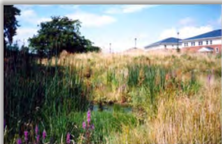
A Stormwater Wetland in Scotland
