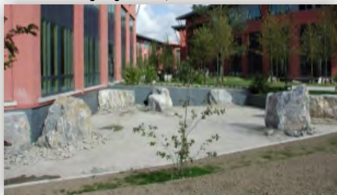
Dry Detention Basin, South Dublin
