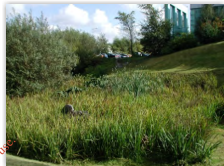
Vegetated Detention Basin
