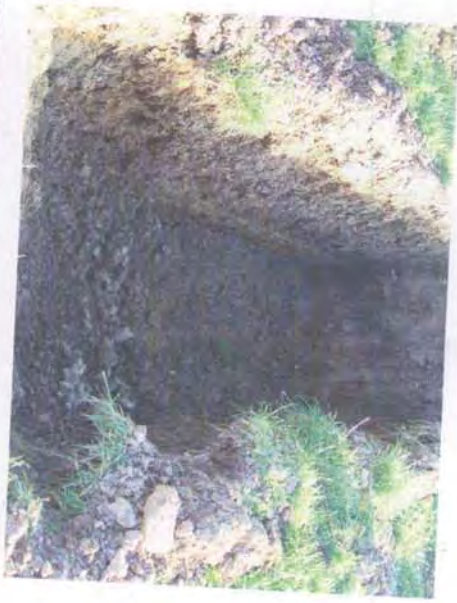
Trial Hole & T-Test Hole
