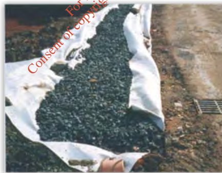
A Filter Drain under Construction
