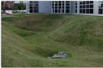
Grassed Detention Basin, South Dublin
