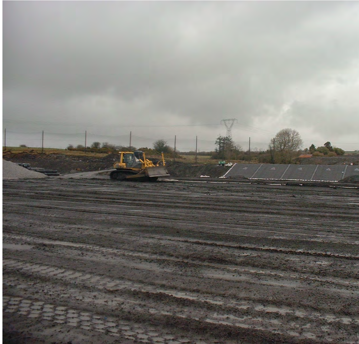
Construction of Waste Cell to Formation Level
