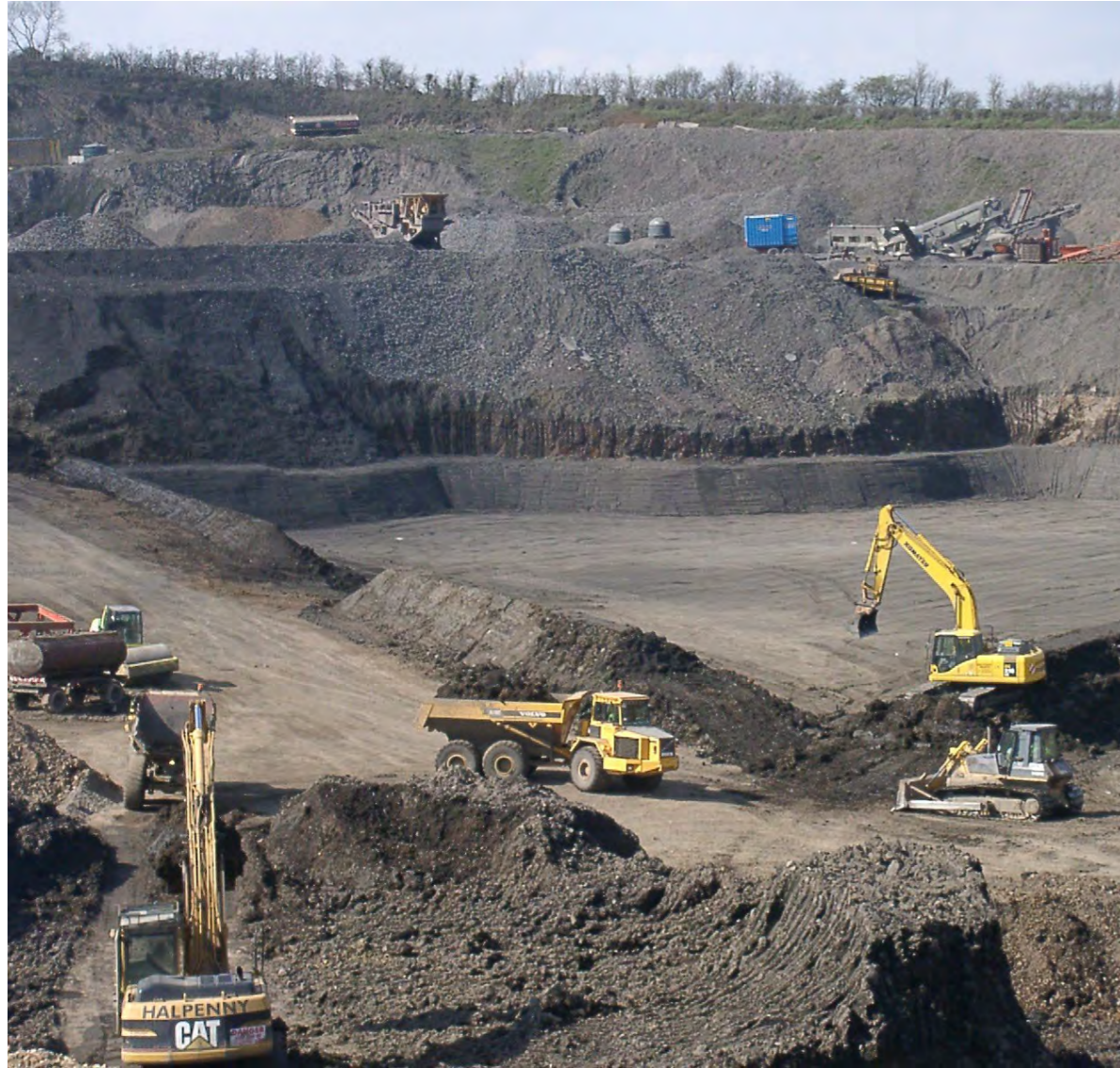
Construction of Inert Cell with Clay Liner
