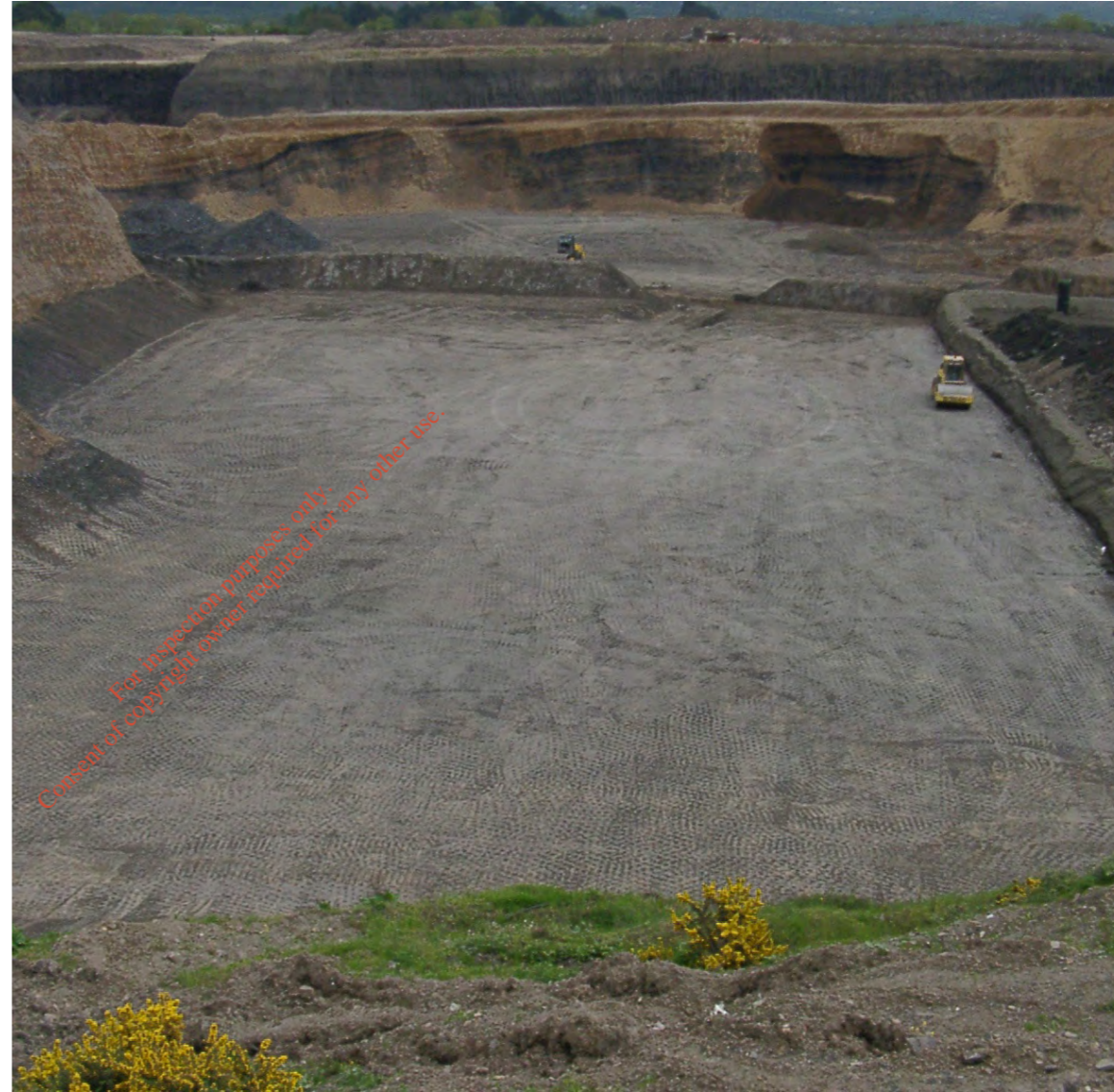
Construction of Inert Liner on Base of Waste Cell
