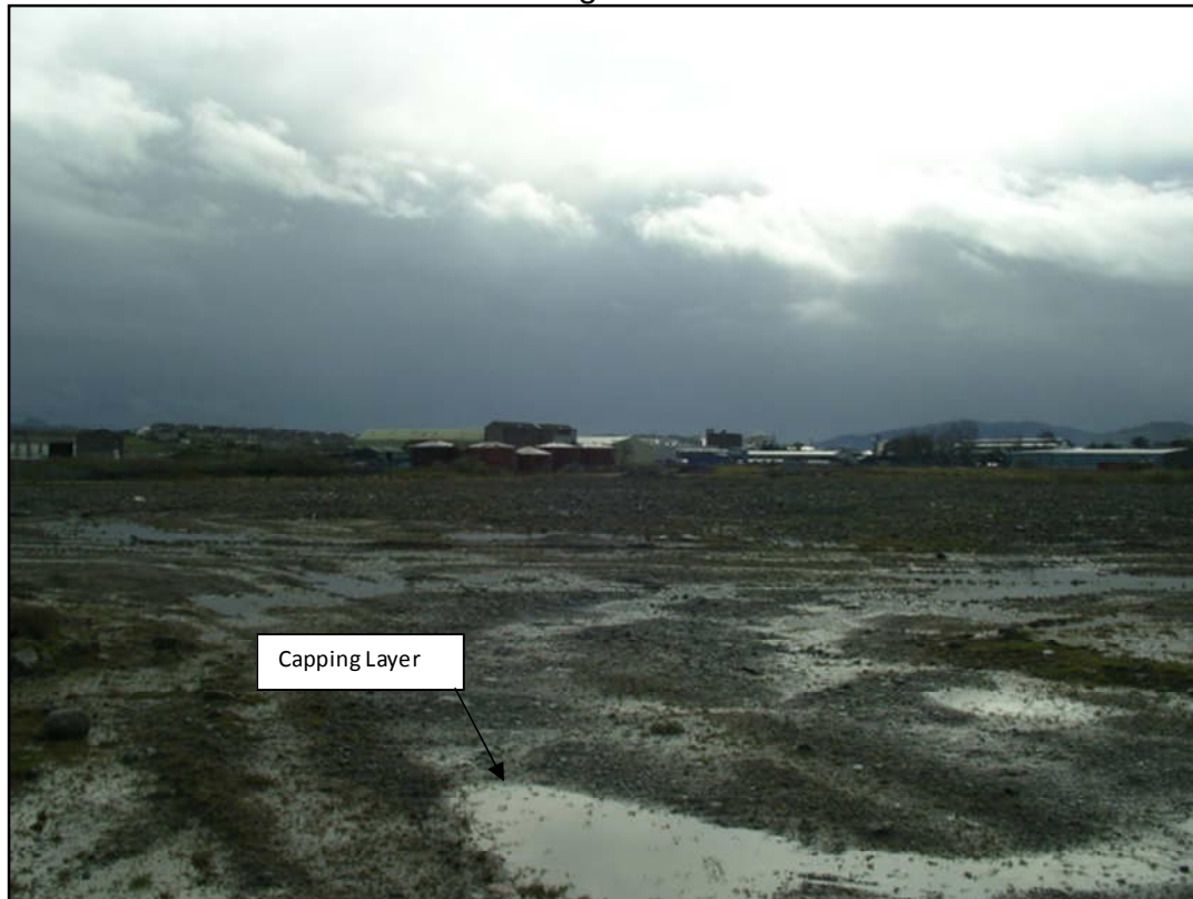
Photograph 7: View looking east. Please note capping layer/material in foreground.
