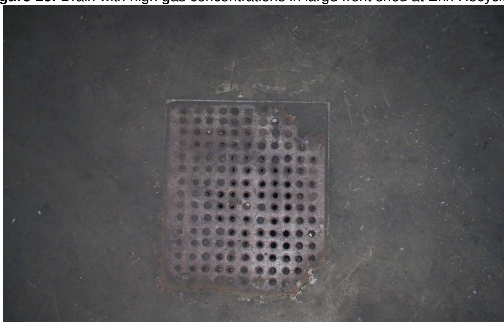
Figure 16: Drain with high gas concentrations in large front shed at Erin Recyclers.
