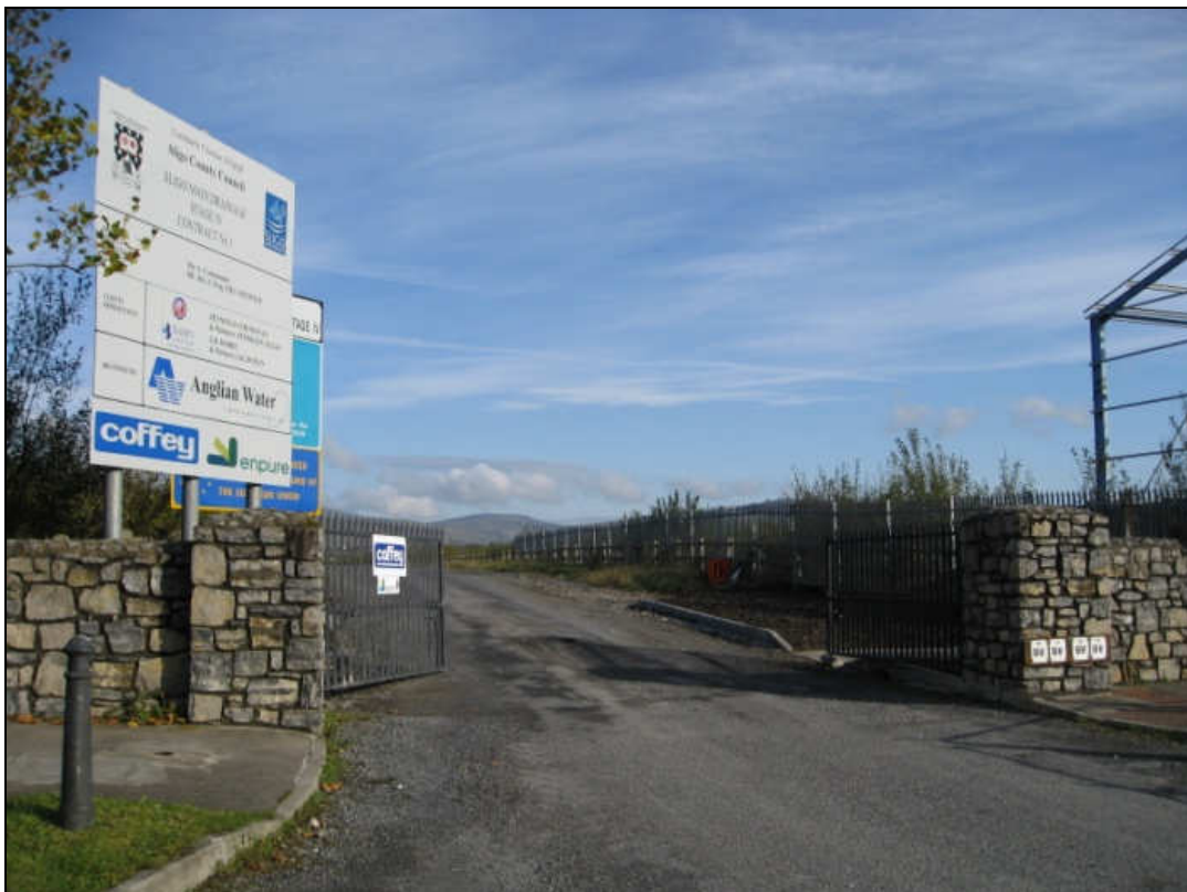
Photograph 12: View looking north east at the main entrance to the WWTP located off Finisklin road
