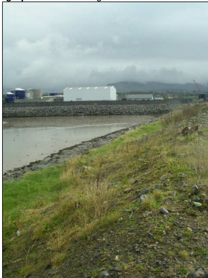
Photograph 2: View looking north east towards the WWTP
