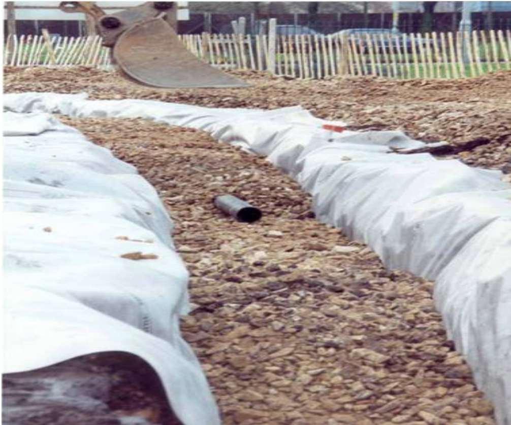
Backfilling the geotextile lined vent trench with coarse aggregate; horizontal gas collection pipe being installed
