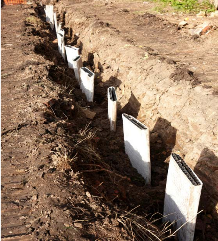
Vertical vent nodes that form a key part of the Virtual Curtain System
