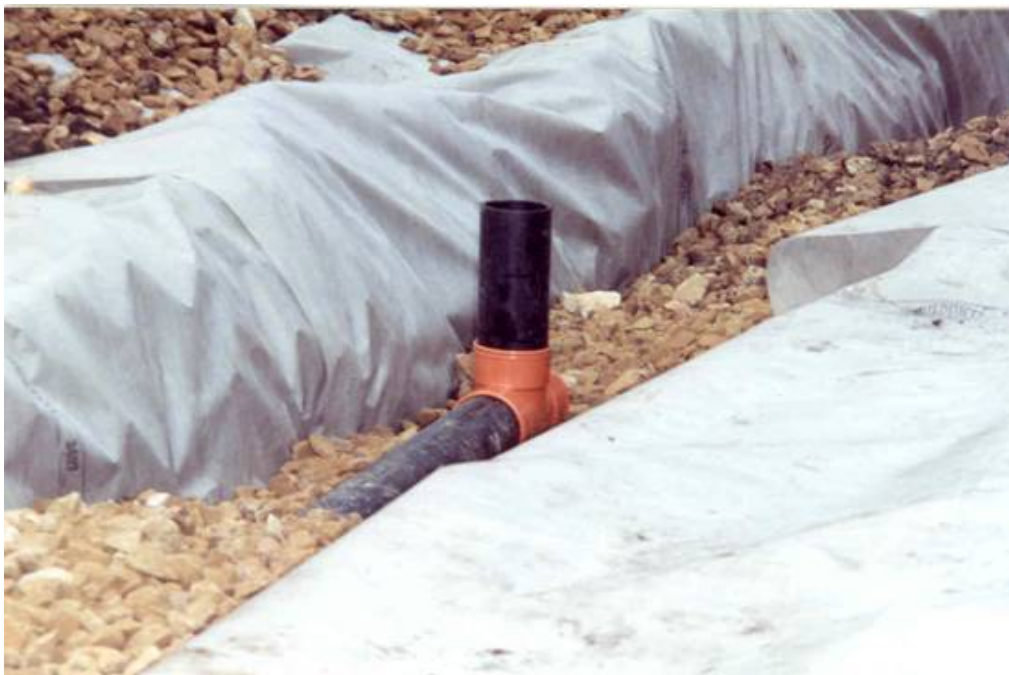
Connection of horizontal gas collection pipe to vertical vent stack
