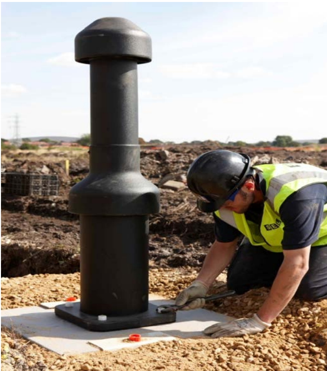
Vertical vent bollards
