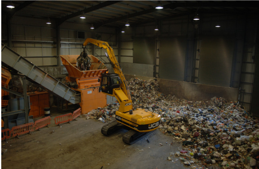
Typical Mechanical Grab Machine in Operation Typical Waste Presorting
