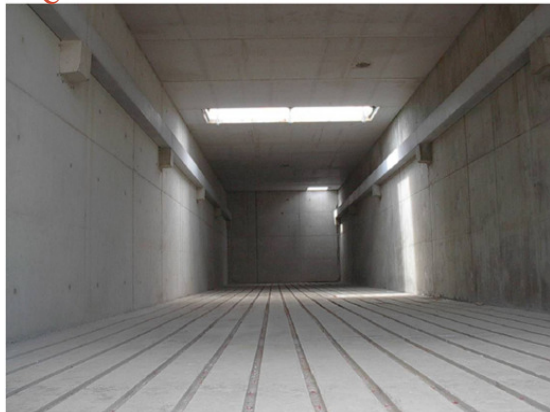
Typical Composting Tunnel with Spigot Floor
