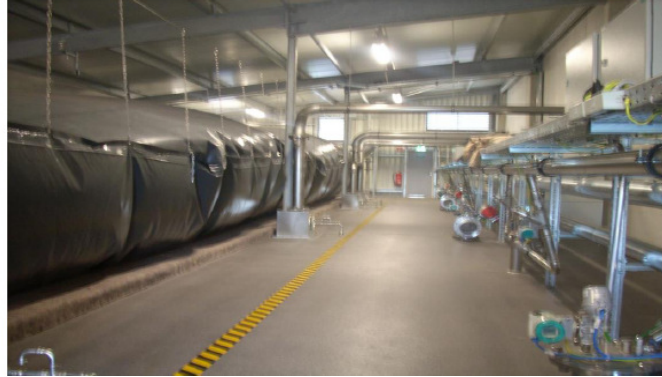
Typical Biogas Storage Units
