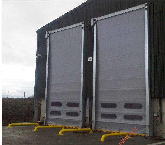
Typical Waste Receiving Doors
