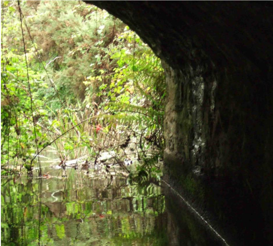
Plate 7 Tramore River: Site E - view of kick-sample site under bridge (23-09-2011)
