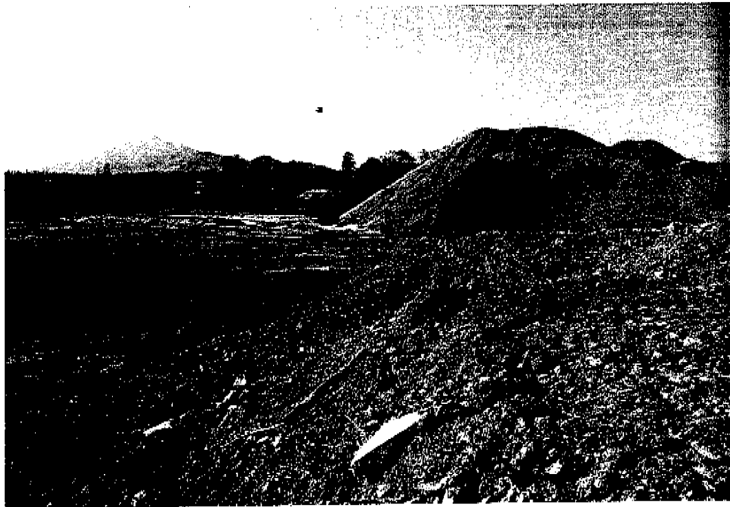
Plate 2 : View Southwards across Existing Backfilled Slope
