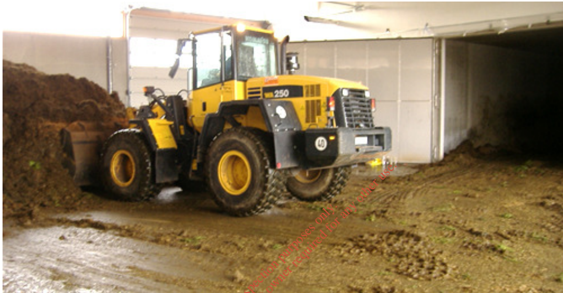
Figure 5 Filling of a fermentation chamber with Bio-waste
