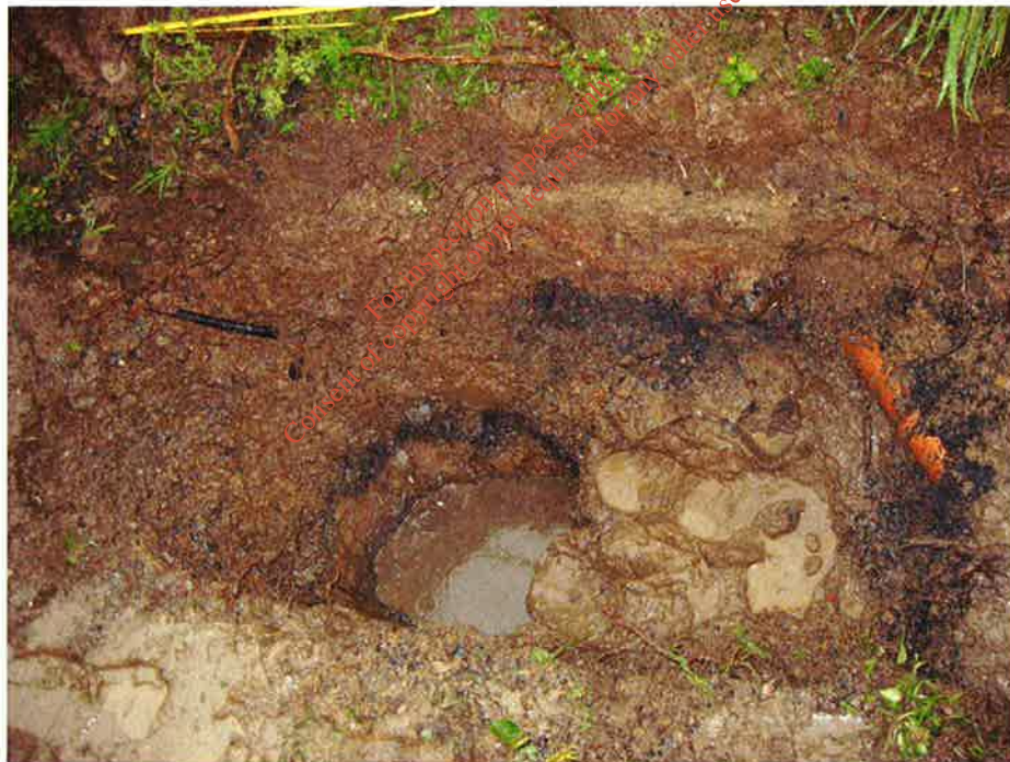
F12 Inspection Pit
