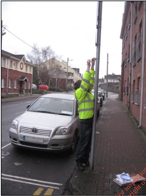
Plate 1: Site 1, View 1 - St Alphonsus Street
