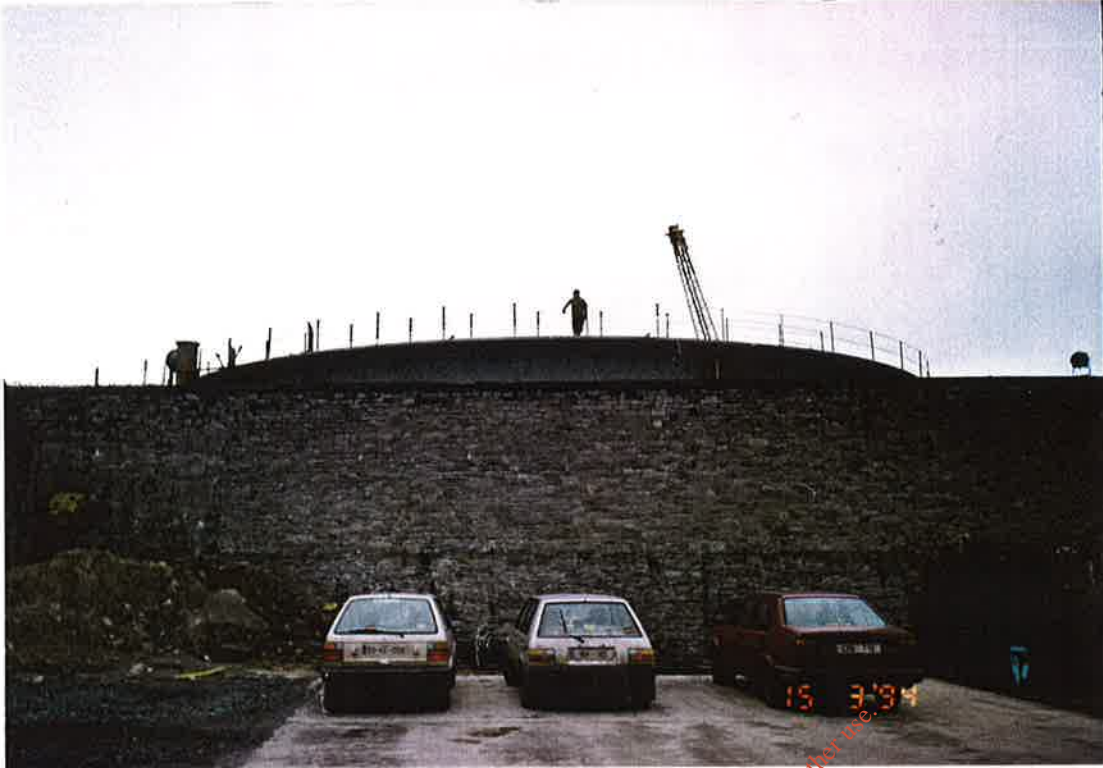
LIMERICK SITE PROGRESS PHOTOGRAPH NUMBER 3.
