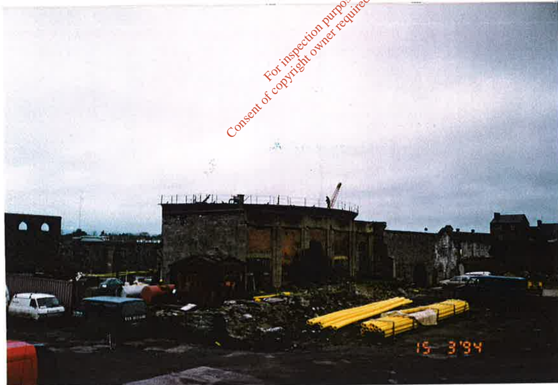
LIMERICK SITE PROGRESS PHOTOGRAPH NUMBER 4.
