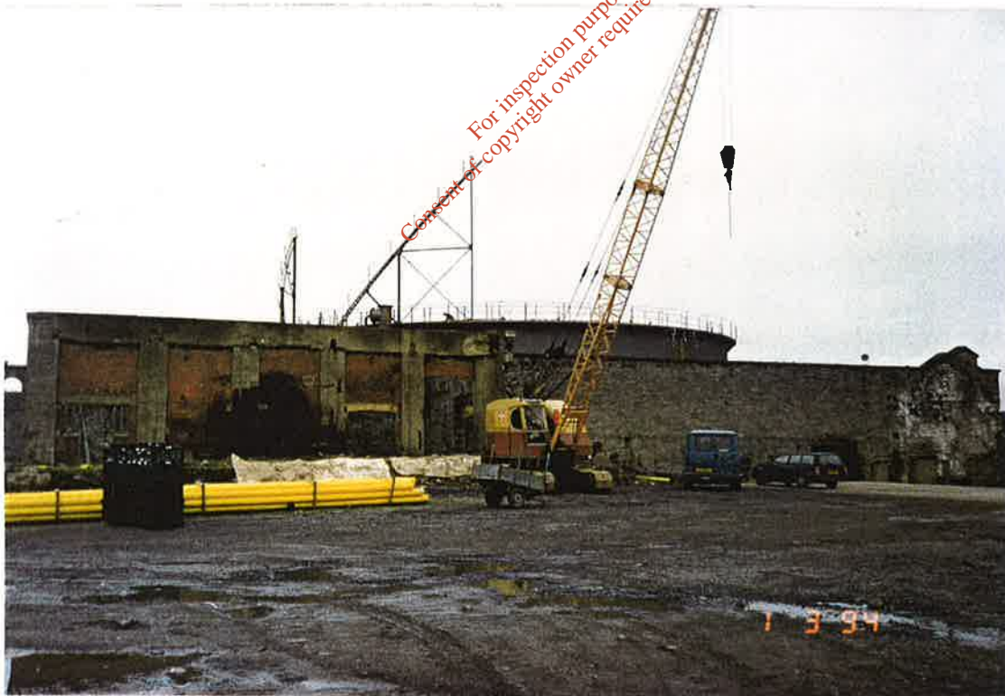
LIMERICK SITE PROGRESS PHOTOGRAPH NUMBER 2.
