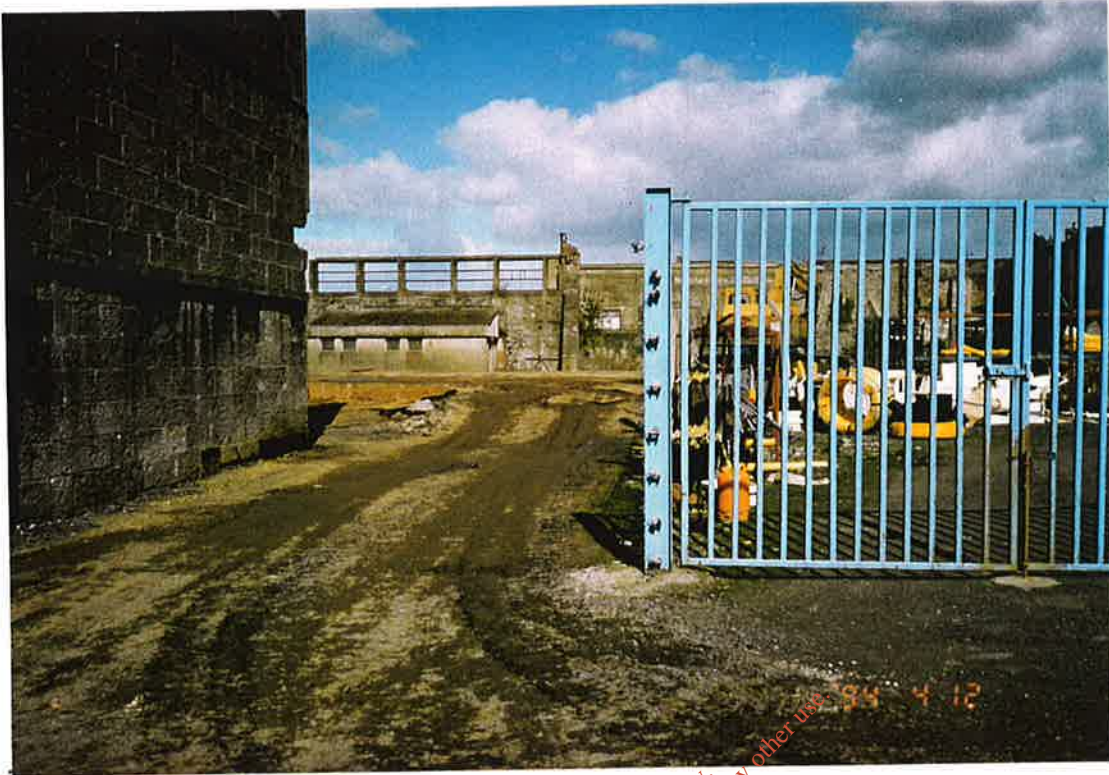
LIMERICK SITE PROGRESS PHOTOGRAPH NUMBER 7.
