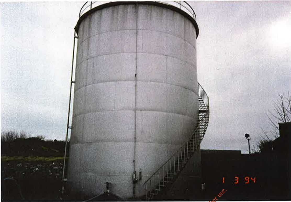
LIMERICK SITE PROGRESS PHOTOGRAPH NUMBER 1.
