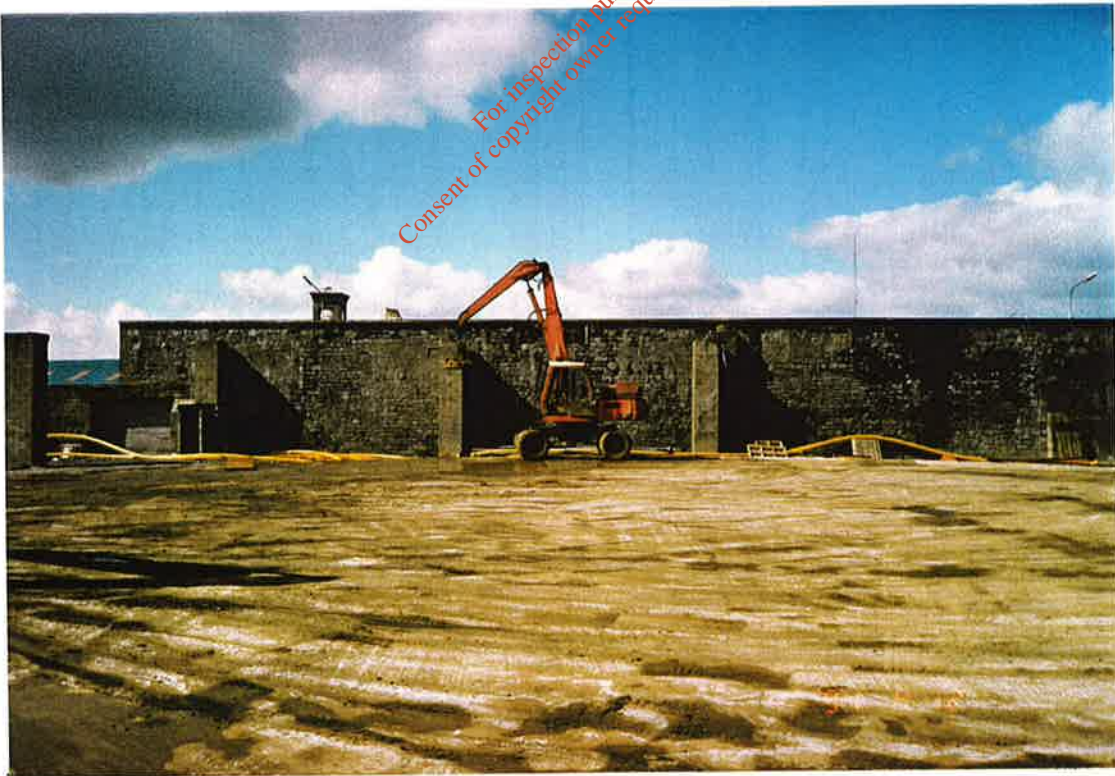
LIMERICK SITE PROGRESS PHOTOGRAPH NUMBER 8.
