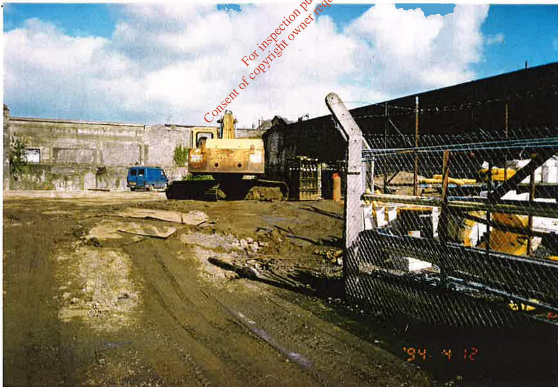
LIMERICK SITE PROGRESS PHOTOGRAPH NUMBER 6.
