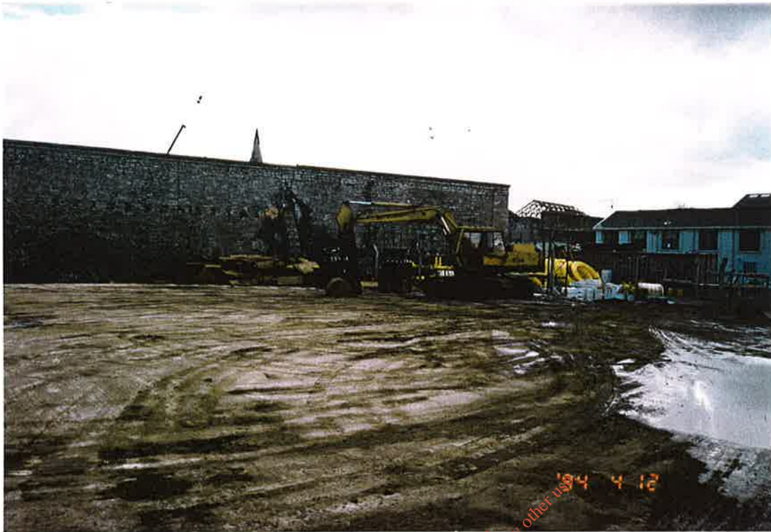
LIMERICK SITE PROGRESS PHOTOGRAPH NUMBER 5.
