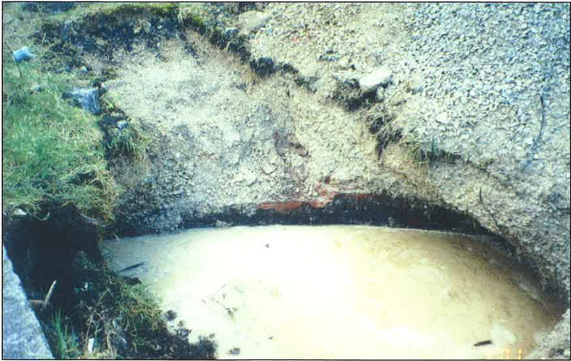
TP 37 View North Showing Brick Tank Wall
