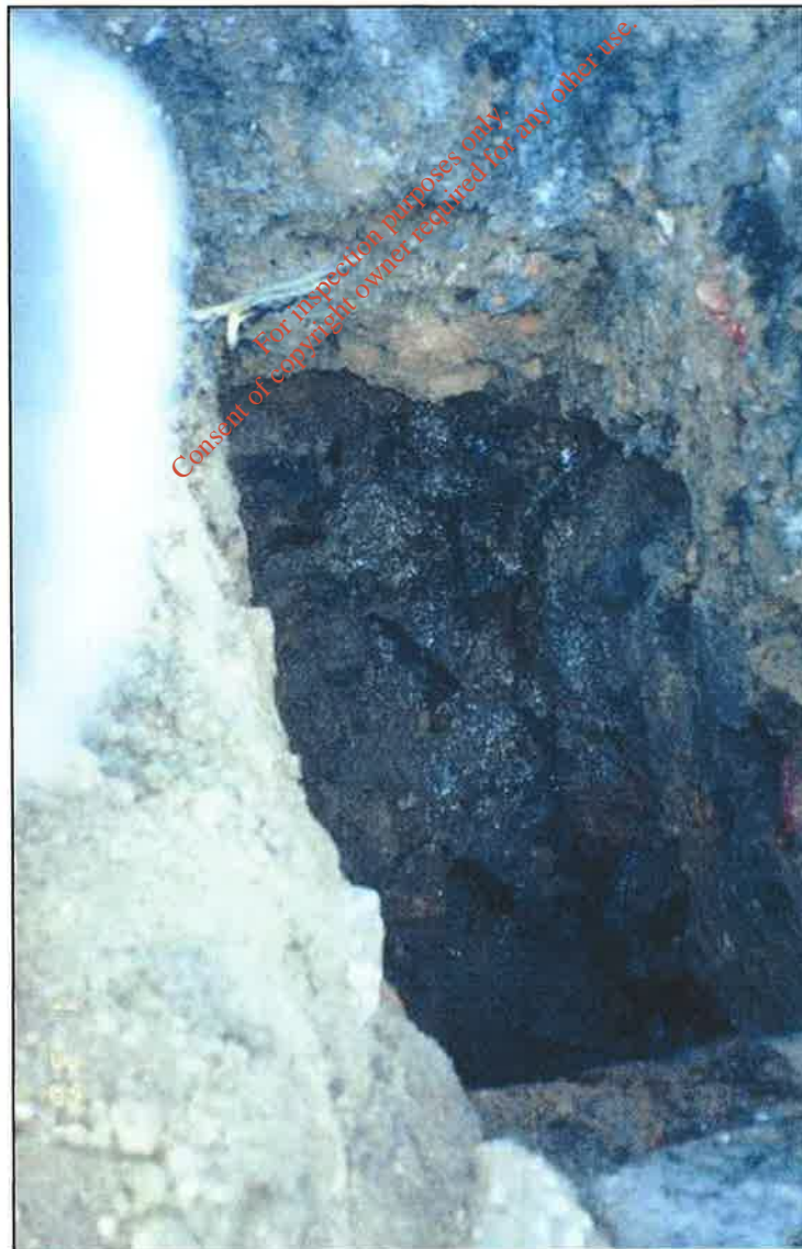
TP 48B View into Contents of Tank
