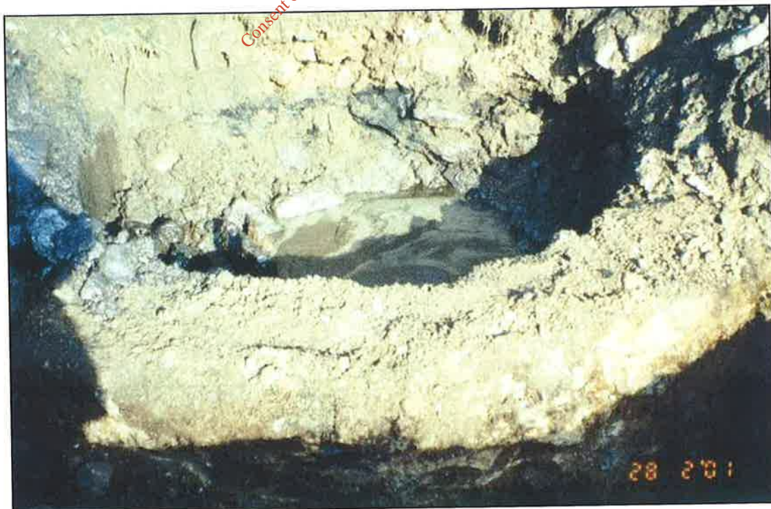
TP 49 View East of Wall
