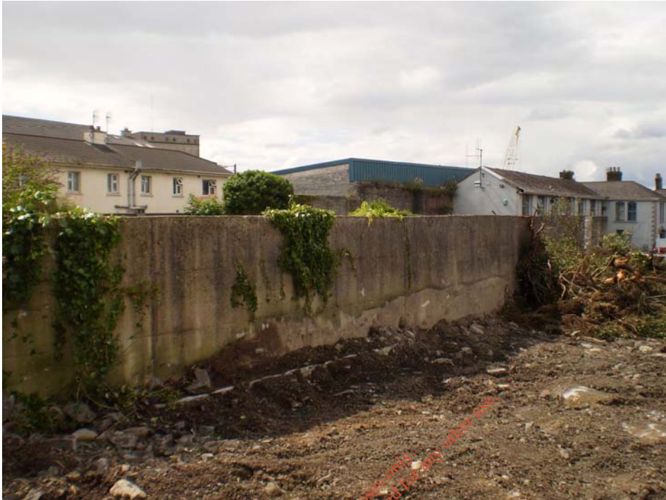
Photo 39) Tank 1 bund exterior
