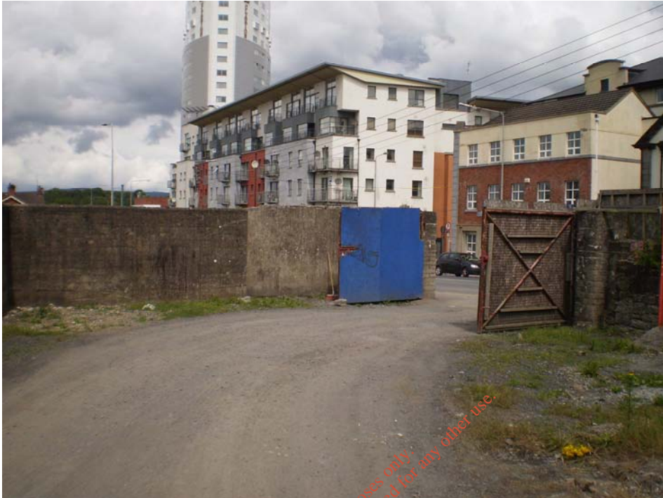
Photo 25) O' Curry St site entrance
