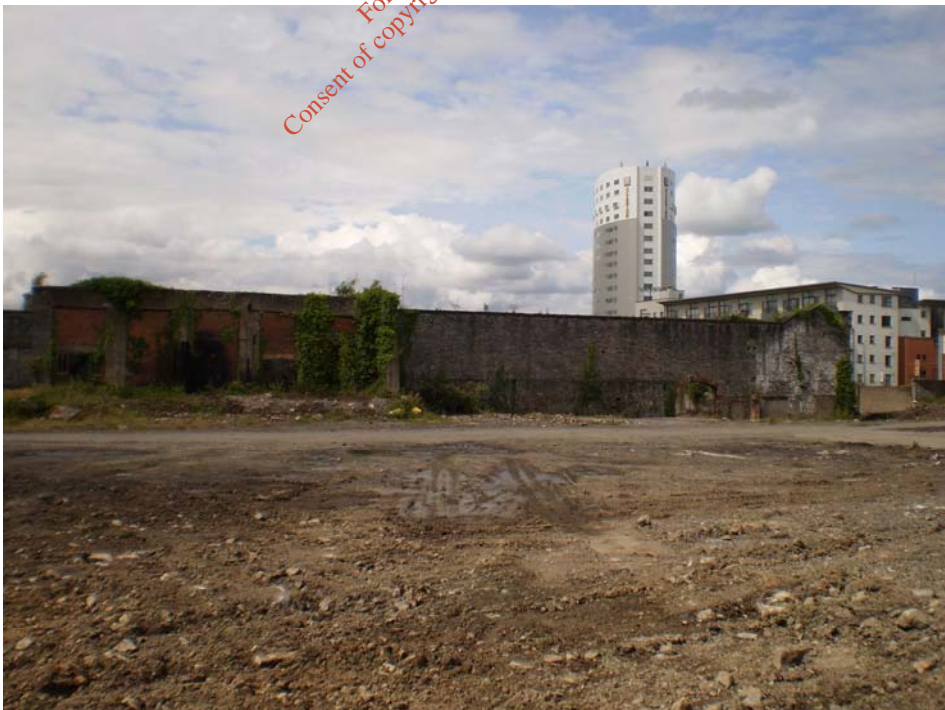
Photo 40) View west across the site
