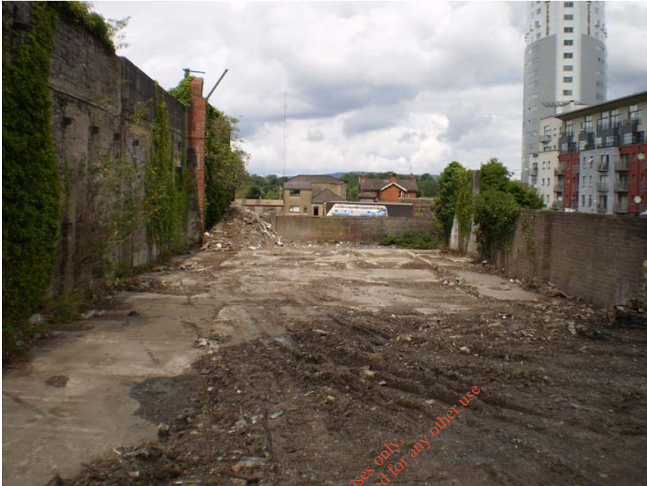
Photo 21) View towards Gasholder 1
