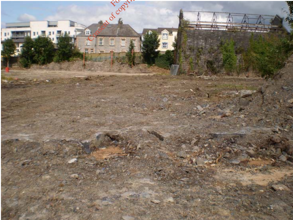
Photo 38) Exposed limestone bedrock
