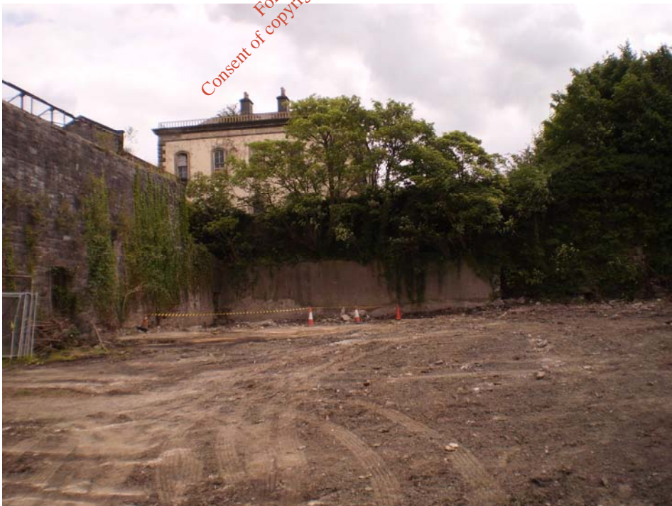
Photo 32) South west side of No.5 stores
