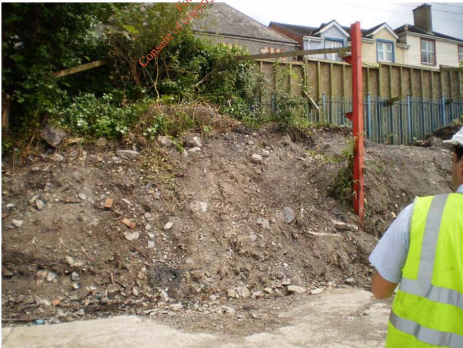
Photo 28) North eastern boundary
