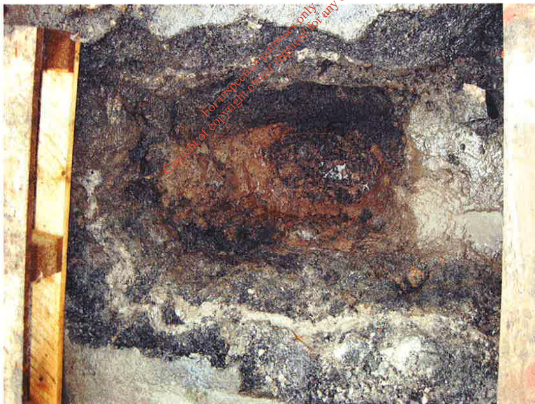
C11 Inspection Pit
