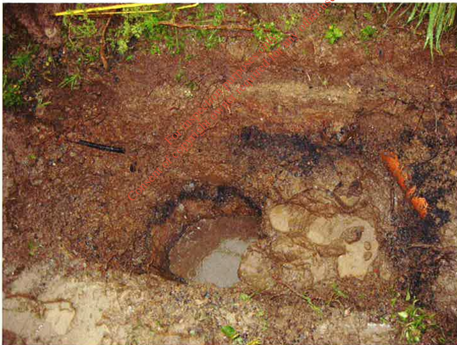
F12 Inspection Pit
