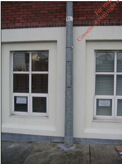
Plate 13: Site 4, View 2 – O'Curry Street
