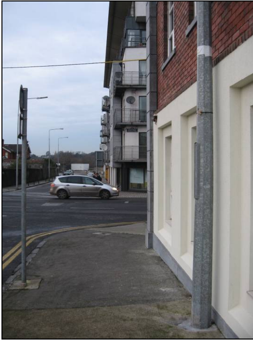
Plate 12: Site 4, View 1 – O'Curry Street
