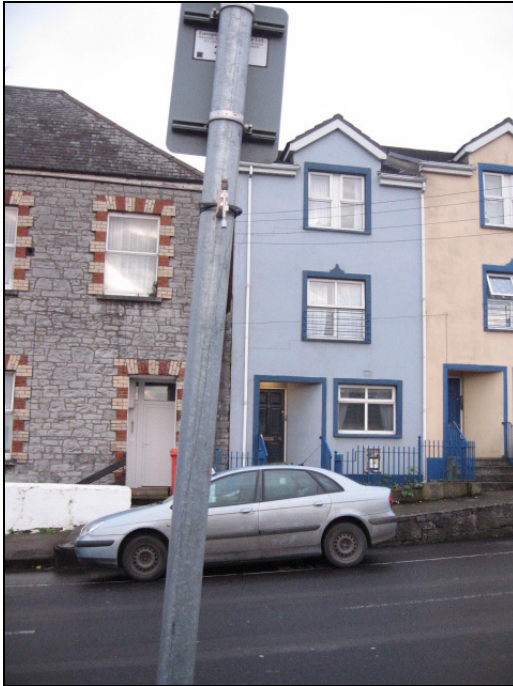
Plate 8: Site 3, View 1 – O’Curry Street
