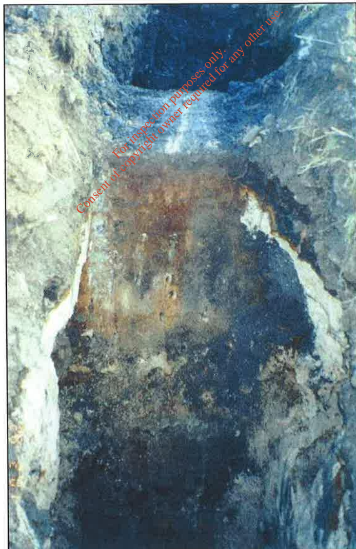
TP 35 Looking North at Tank Wall
