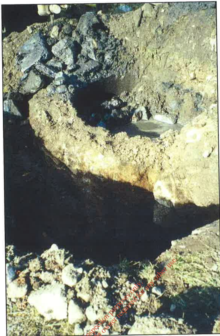
TP 49 View North of Wall
