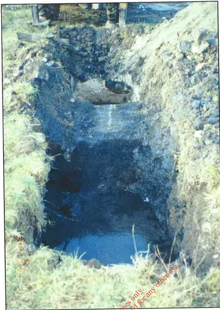
TP 35 Looking South at Tank Wall
