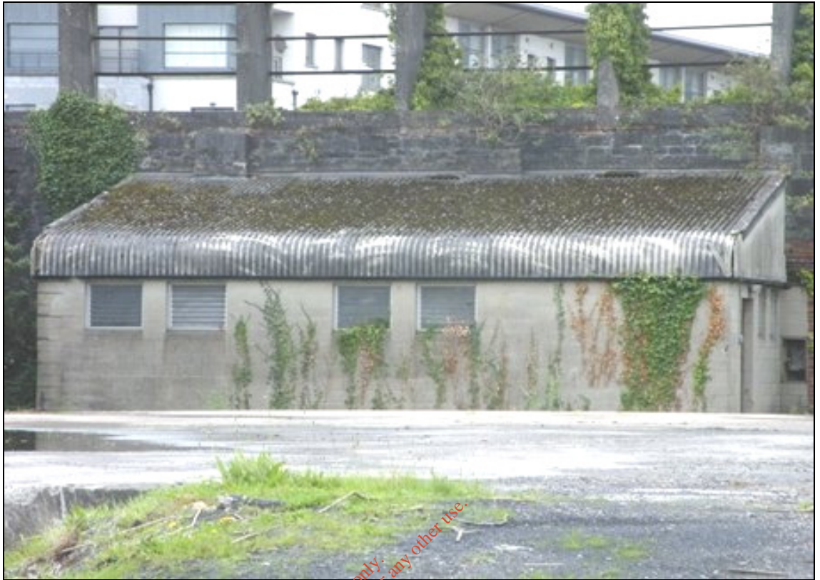
Plate 3: Modern 'lean-to' shed adjoining older walls at north of site
