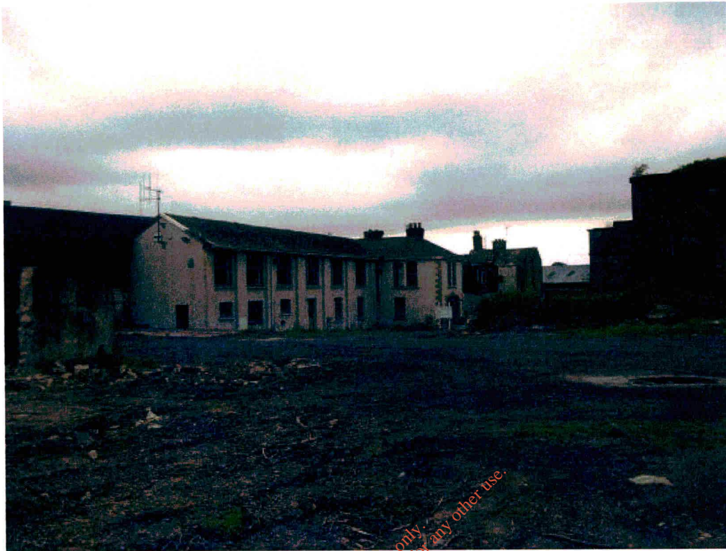
Photo 3 Disturbed ground and the recently vacated offices.
