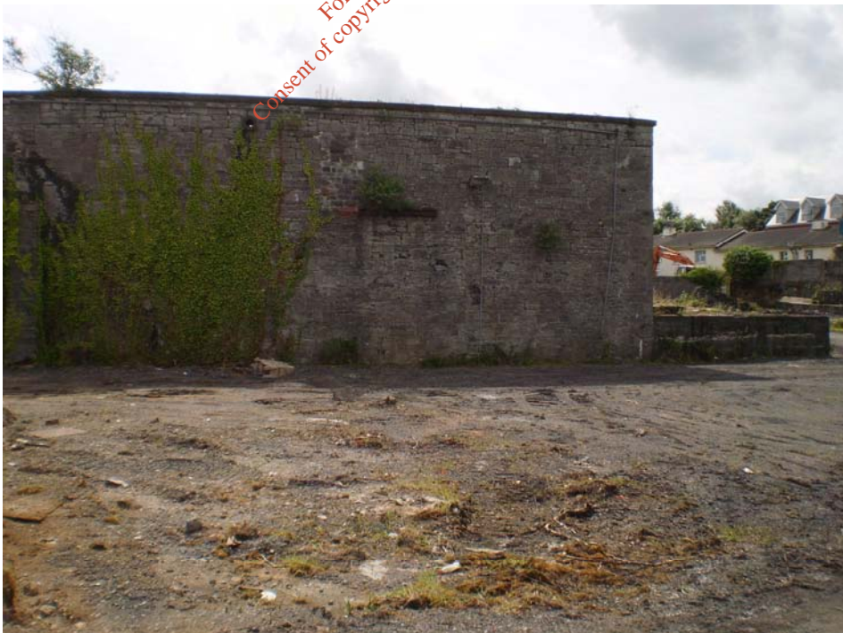
Photo 4) Back wall of booster house
