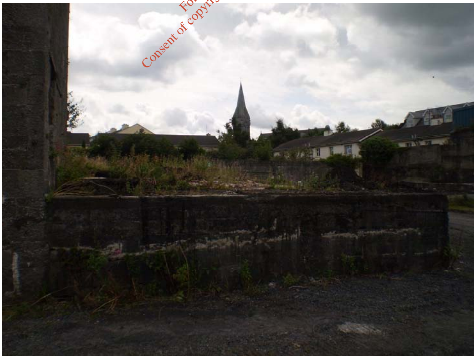
Photo 10) Booster house slab
