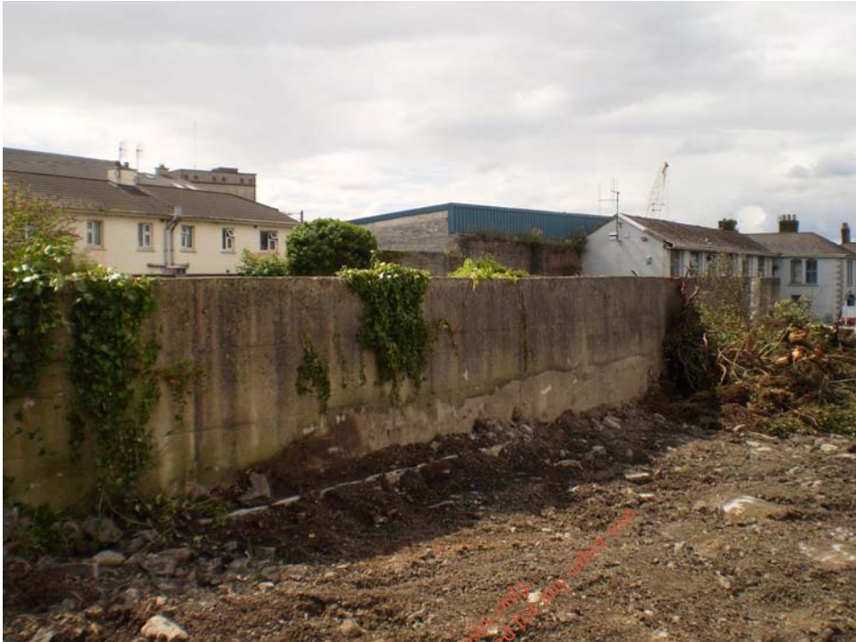
Photo 39) Tank 1 bund exterior
