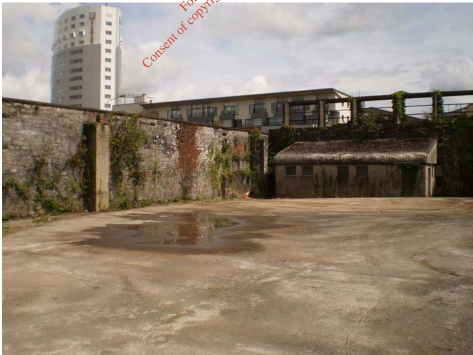
Photo 2) Gasholder 2 and Groverner house
