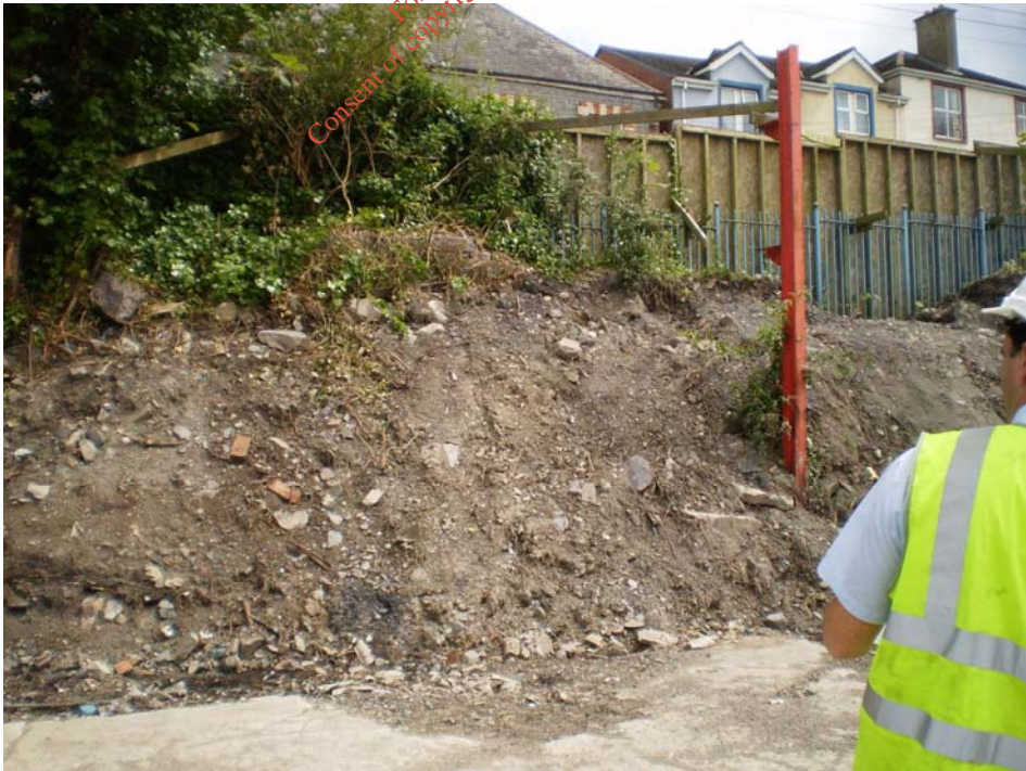
Photo 28) North eastern boundary
