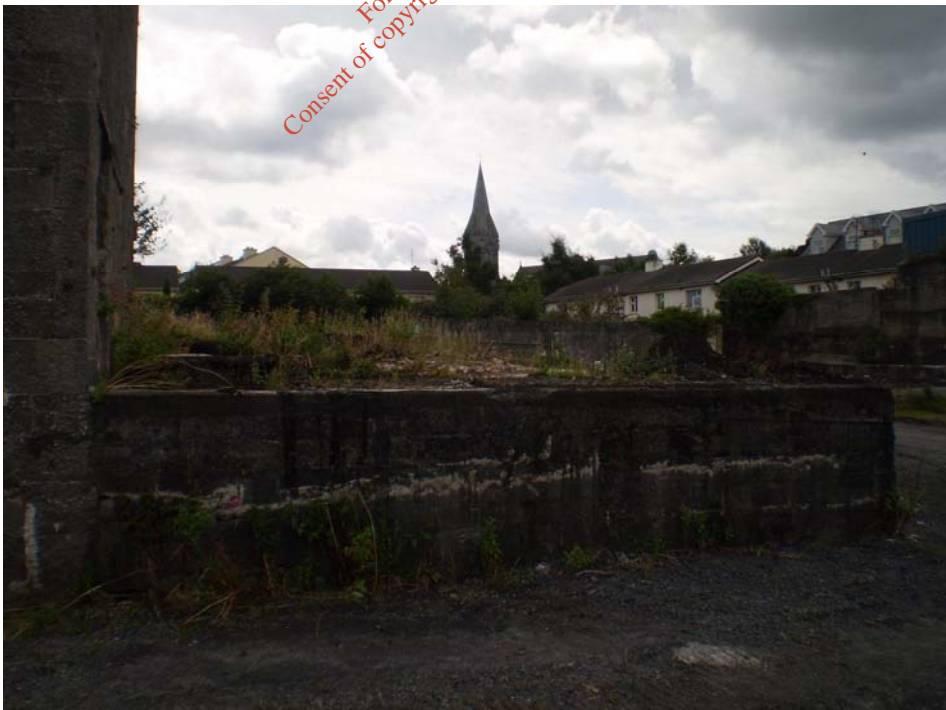
Photo 10) Booster house slab
