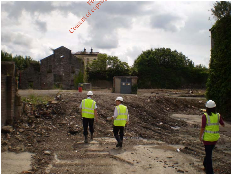
Photo 24) View towards ESB substation
