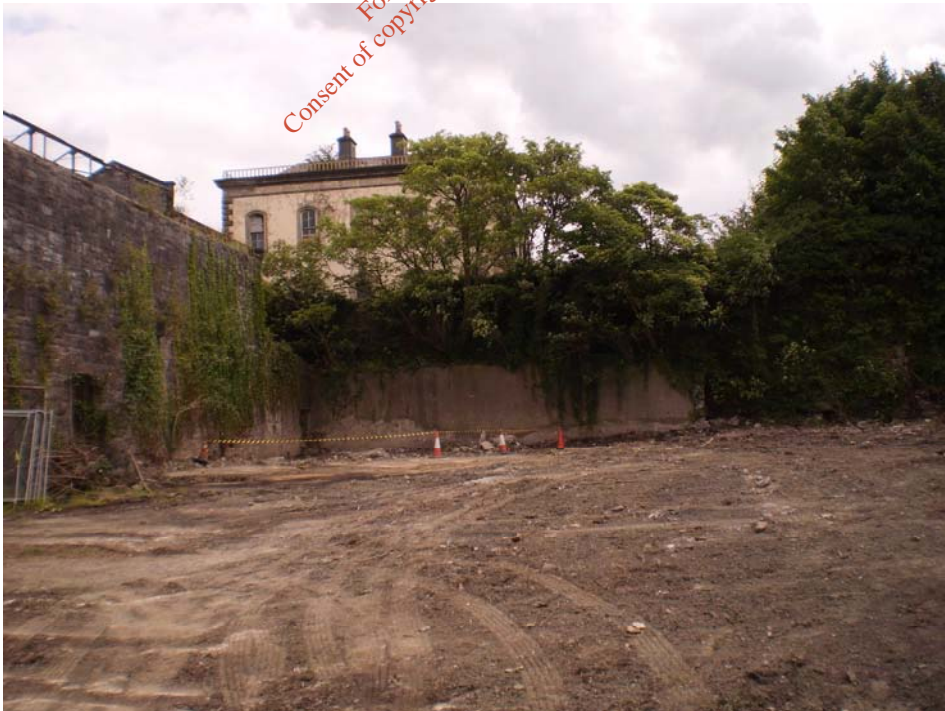
Photo 32) South west side of No.5 stores
