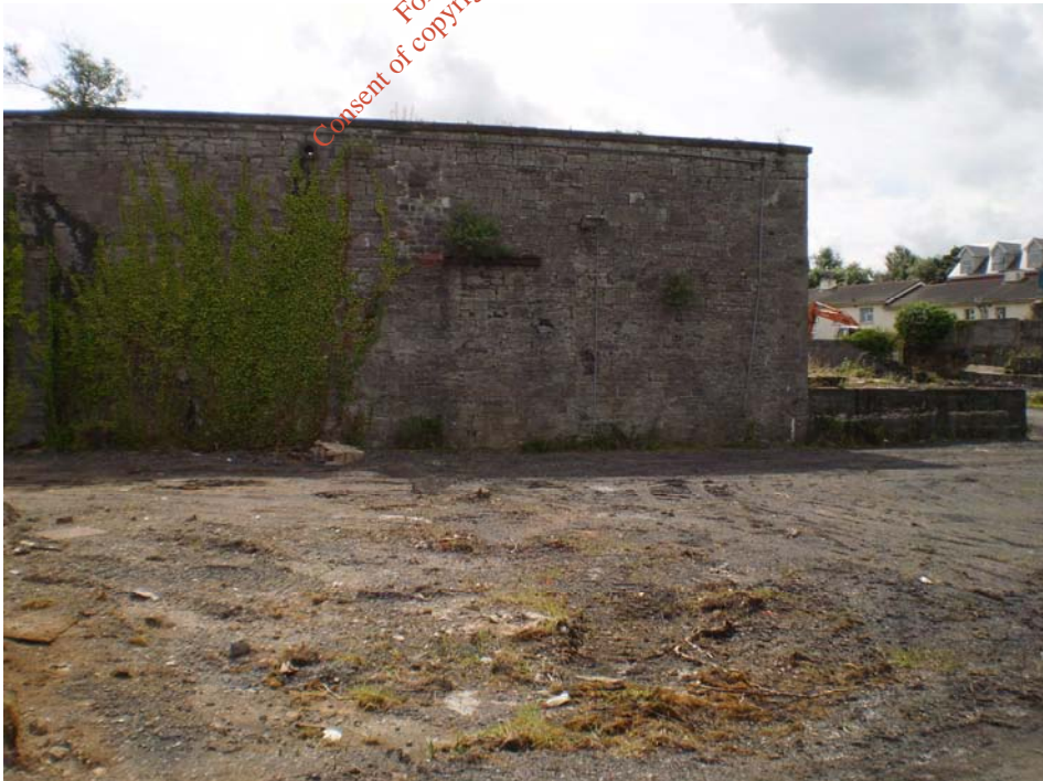
Photo 4) Back wall of booster house
