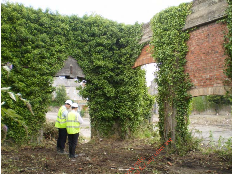
Photo 15) Inside Booster house
