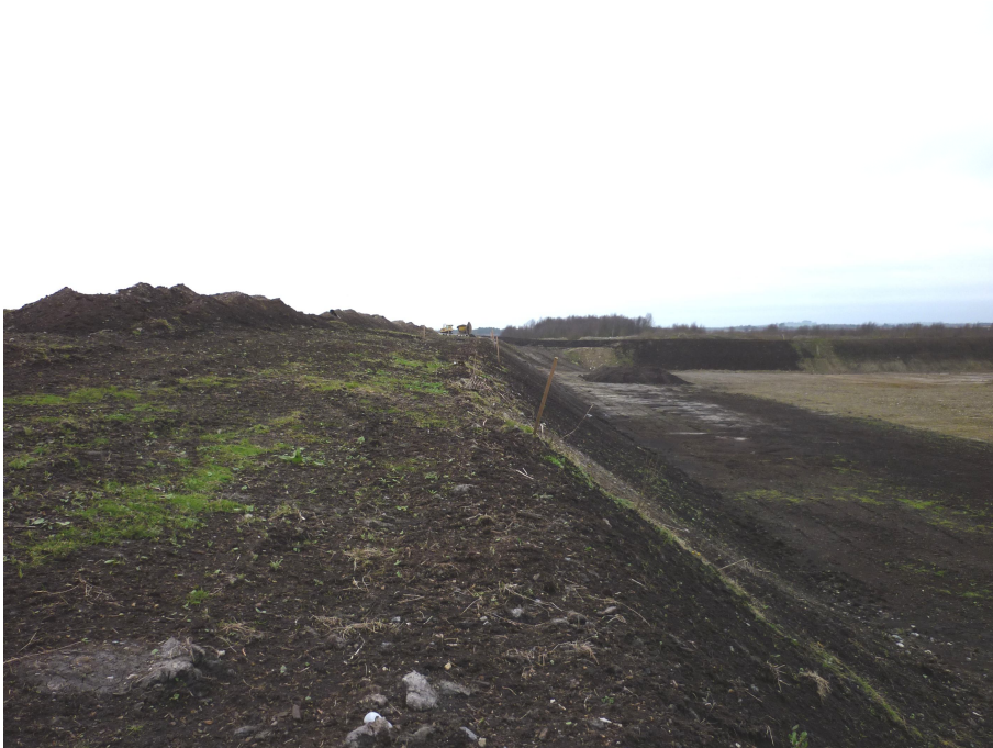
Figure 4 – Cell 2 Northern Embankment
