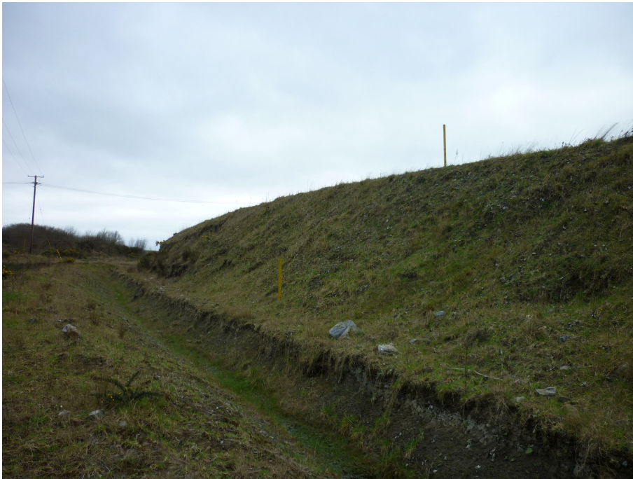
Figure 5 – Cell 3 Southern Embankment
