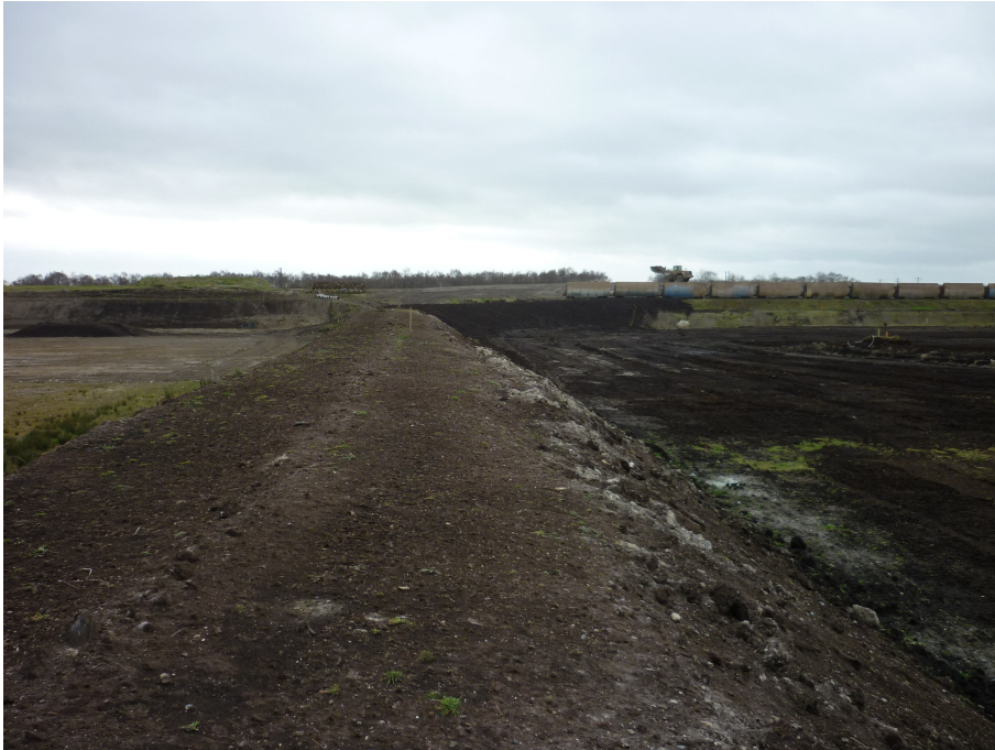
Figure 8 – Cell 4 Eastern Embankment
