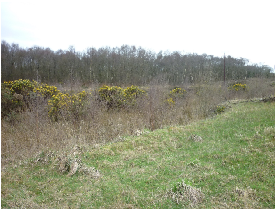
Figure 2 – Cell 2 Southern Embankment
