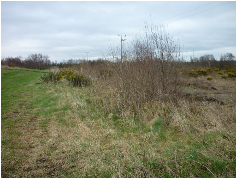
Figure 3 – Cell 2 Southern Embankment
