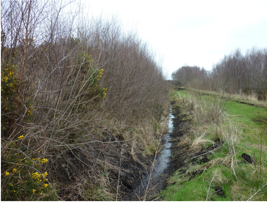
Figure 1 – Cell 1 Eastern Embankment
