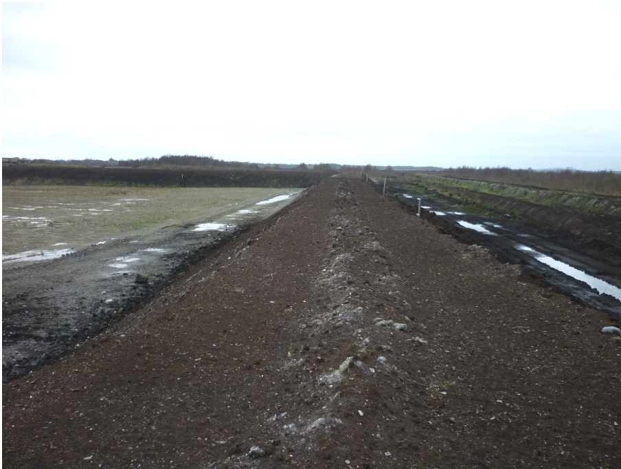
Figure 7 – Cell 4 Southern Embankment
