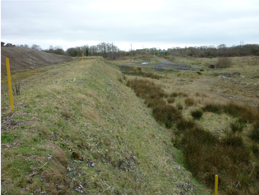
Figure 6 – Cell 3 Western Embankment
