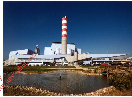
Incinerator in Portugal
