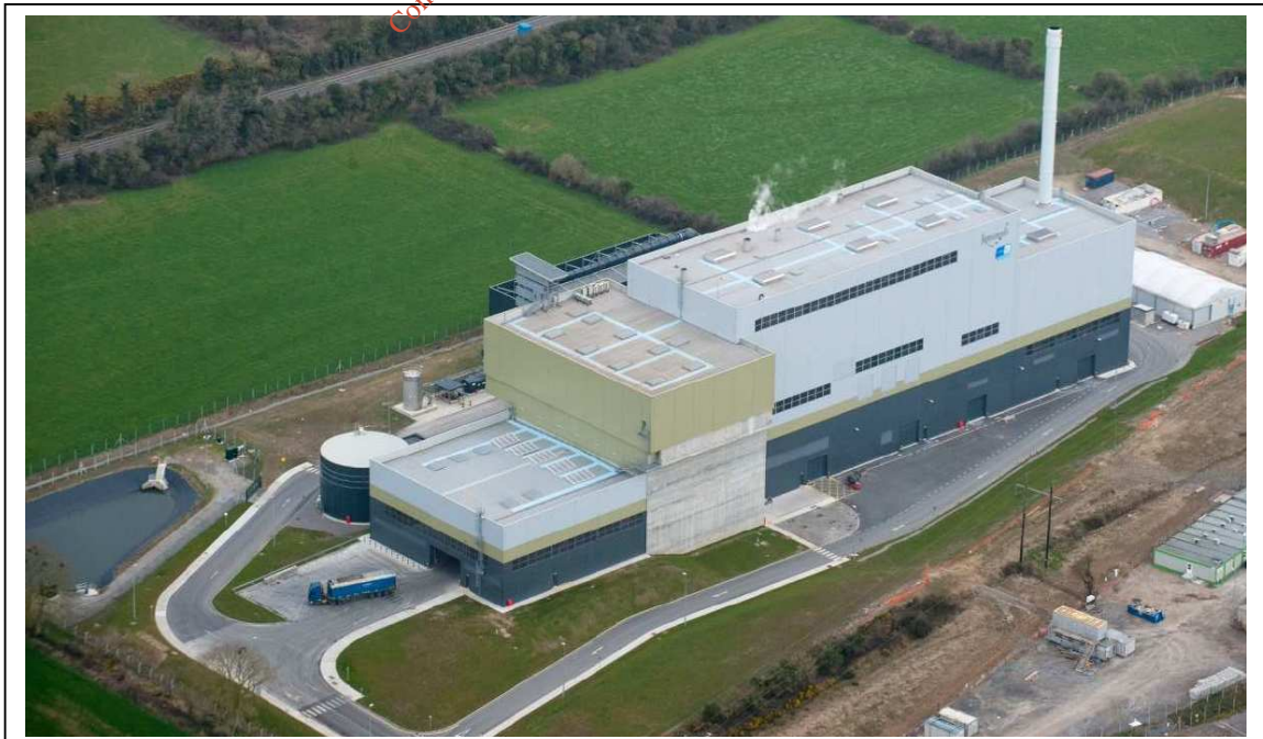
Figure 5.1 Aerial View of Site March 2012
