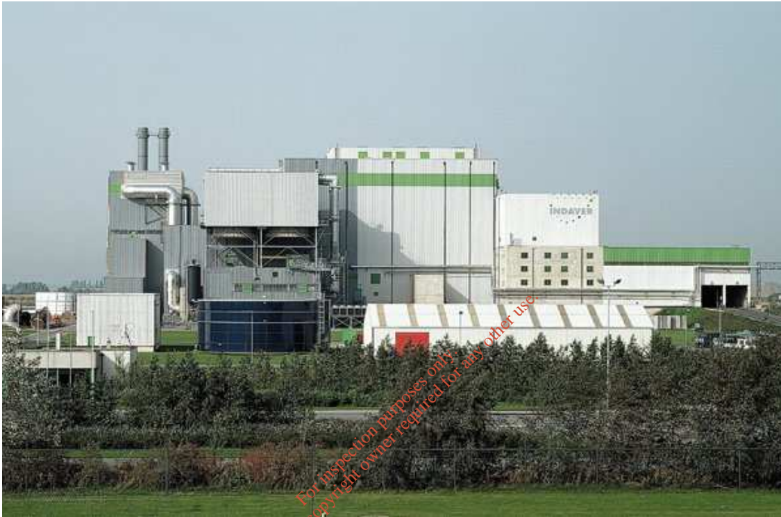
Municipal waste-to-energy facility, Flanders, Belgium
