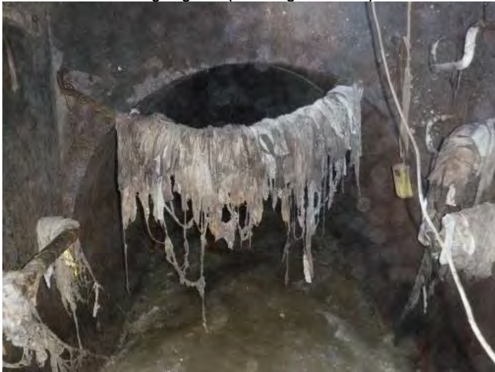
Outgoing flow (Surcharge evidence)
