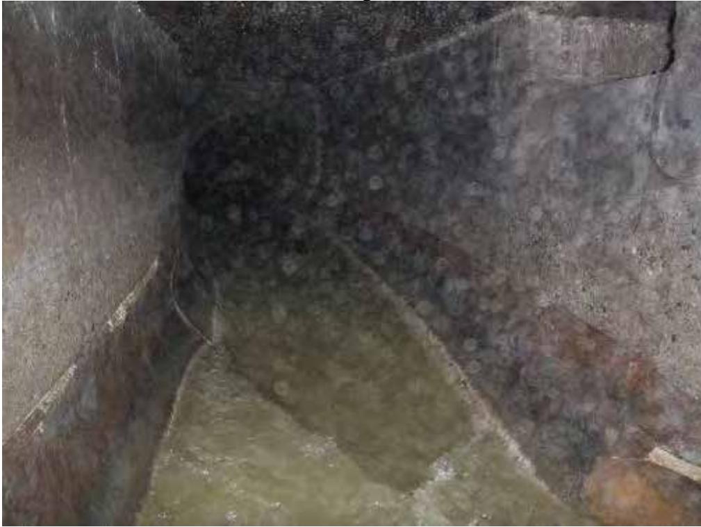
Outgoing flow (Surcharge evidence)
