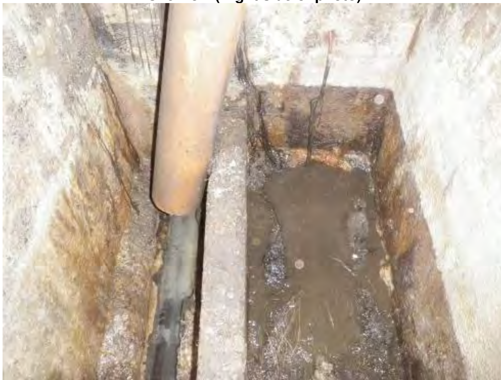
Overflow (Right side of photo)
