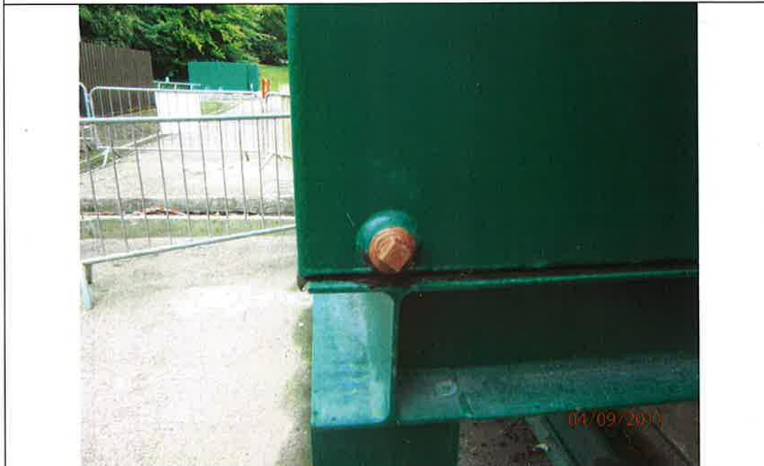
Fig. 39.2: Bund outlet at base for decanting
