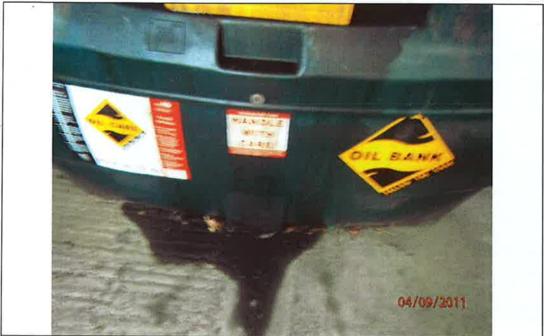
Fig. 38.2: Oil residue from filling (Drip tray required)
