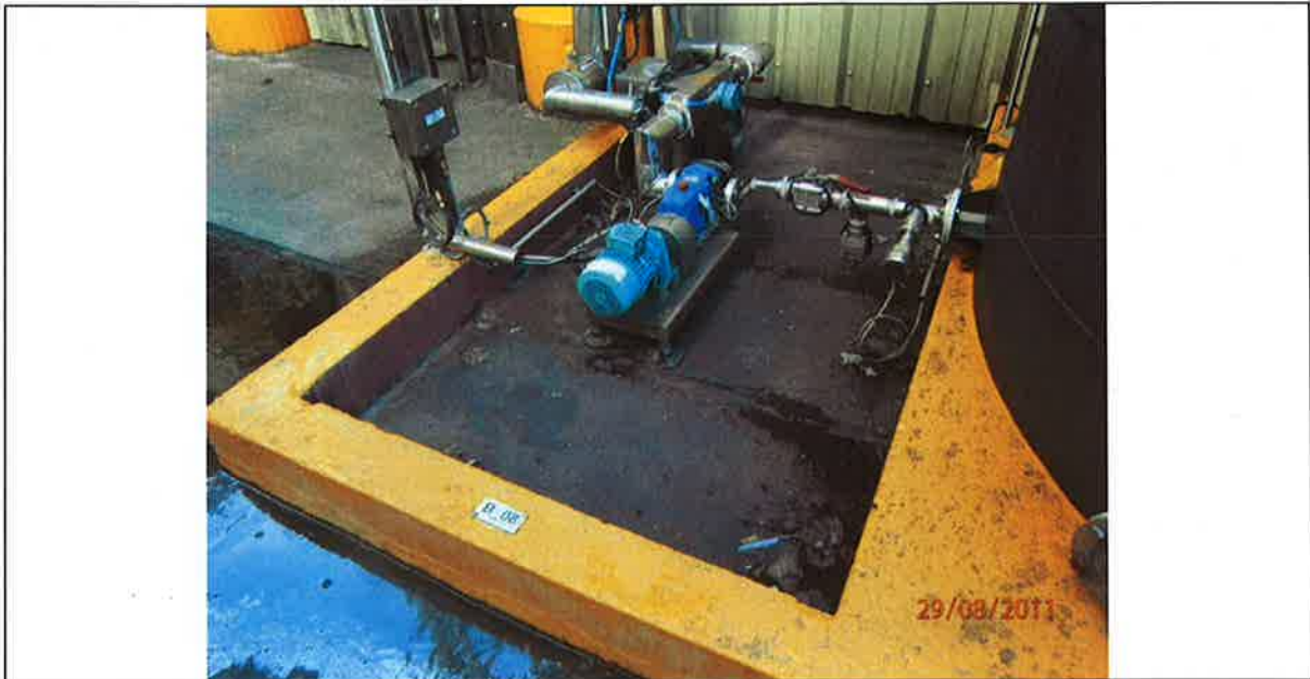
Fig. 8.1: Bund 08 - Bund for pump exiting Bund 07
