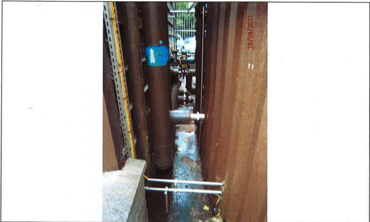
Figure 1.3: Bund 01 – Proximity of CBST1 to east side of bund, limited of access space around tank
