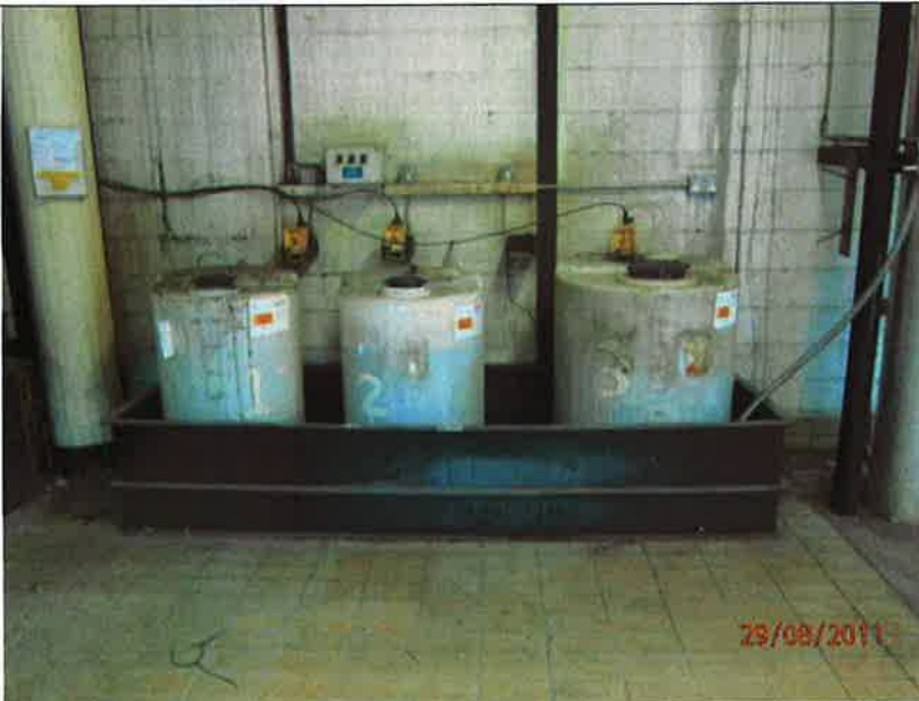
Fig 29.1: Bund 29 - Chemical Additives for Boilers
