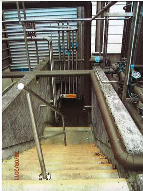
Figure 2.5: Bund 02 – View of underground piping ductway to the west of Bund 02
