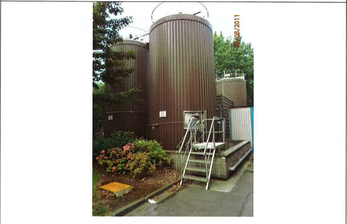
Figure 1.3: Bund 01 – Proximity of CBST1 to east side of bund, limited of access space around tank
