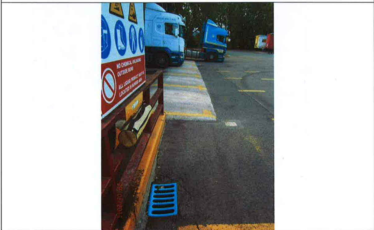
Fig. 6.2 Bund 06 – Surface water drains close to bund
