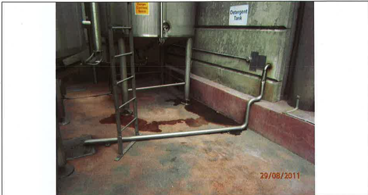
Fig. 17.2: Spill around detergent tank
