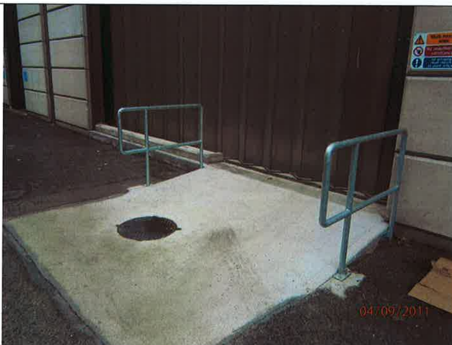
Fig. 32.2: Bund 32 – Kerbing and provision of Aco drains at concertina door
