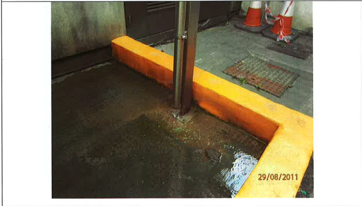
Fig. 20.2: Water draining into Bund 20 from Cooling Towers
