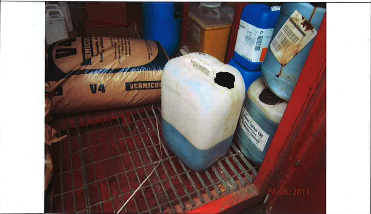
Figure 5.4: Bund 05 – Evidence of haphazard storage in bund container
