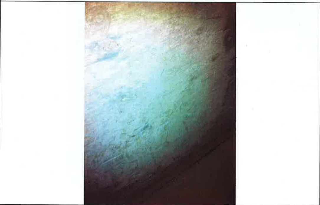
Fig. 41.2: Condition of bund wall
