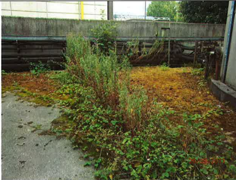
Fig 28.2: Bund 28 – Significant mossy growth and foliage coverage in bund (drainage channel filled with plant growth)
