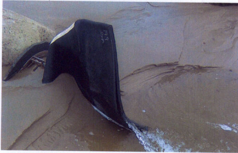
ii. Lower Outfall 09-11-11 – discharging with low sand levels
