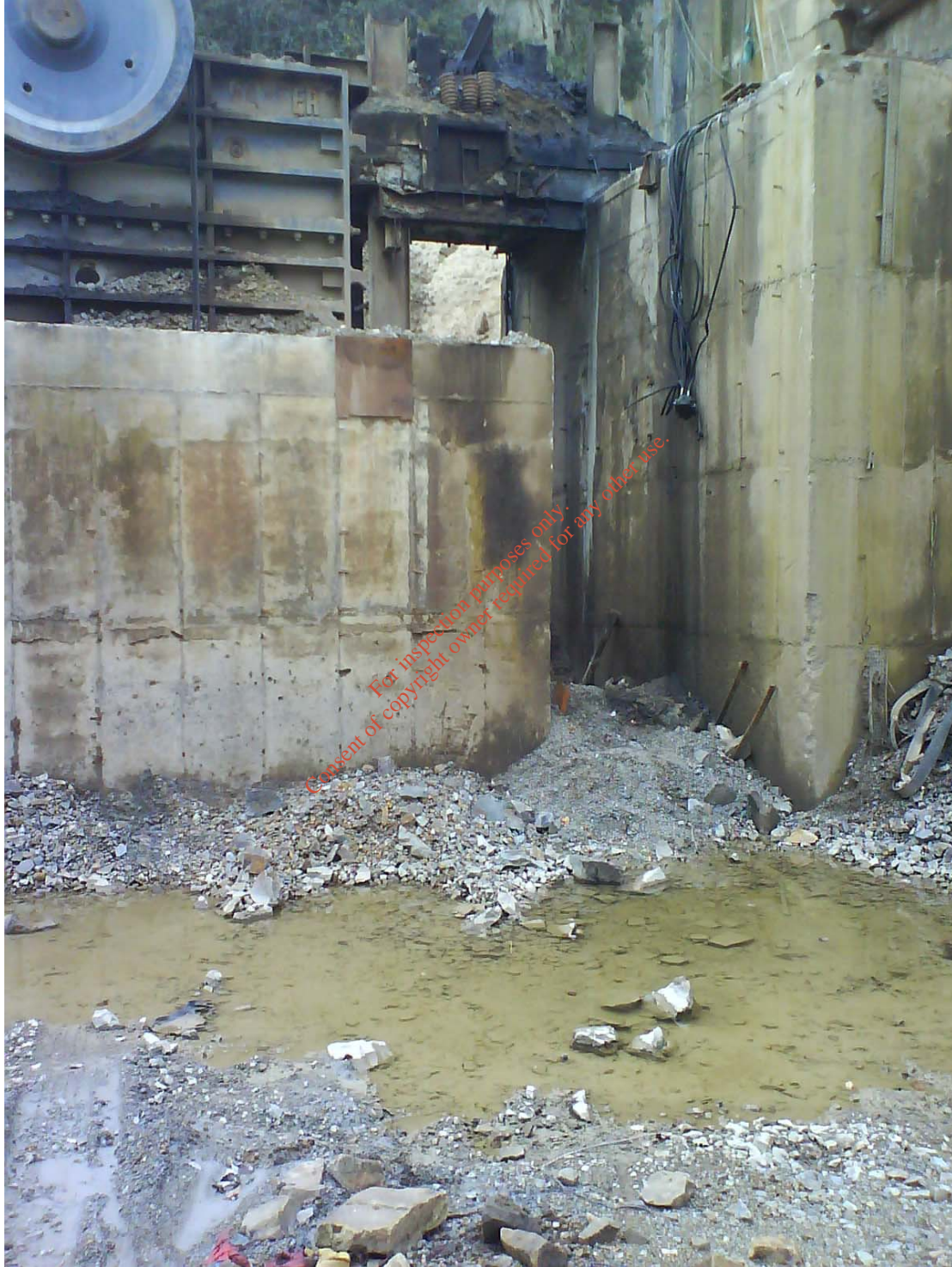
Plate 10: Location of Trial Pit 6 next to dismantled rock breaker
