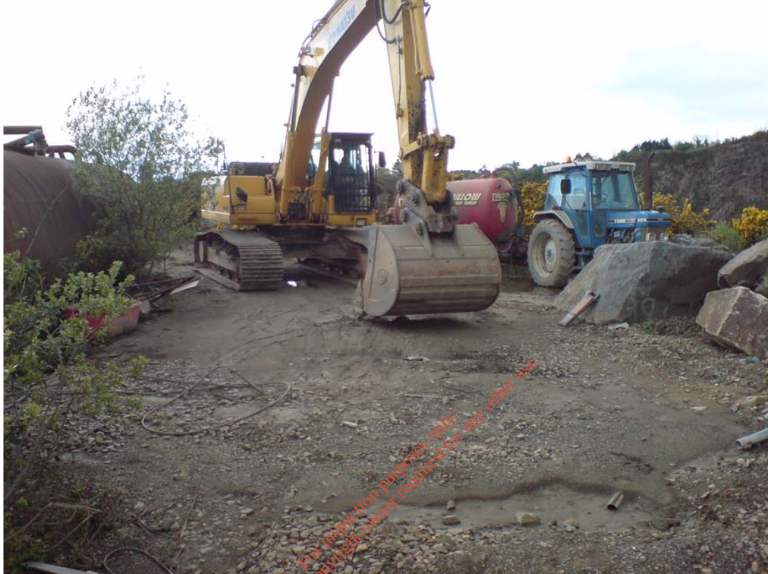
Plate 12: Location of Trial Pit 4
