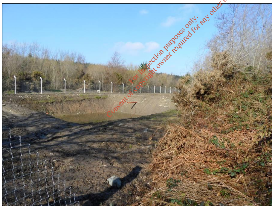
Plate 6 Recently constructed settlement ponds at the south western corner of the Brownswood Quarry site. The surface water from the quarry void will be discharged via a series of these settlement ponds to the cSAC.
