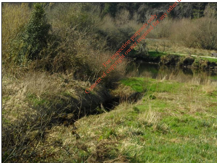
Plate 20 One of many drainage channels which intersect the floodplain between the N11 and the river corridor. These were characteristically overgrown and silted.
