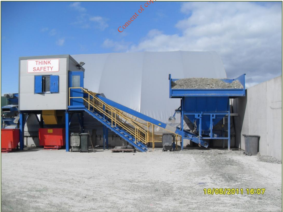
Photograph D.2.8: Hopper and picking station at Drying Plant
