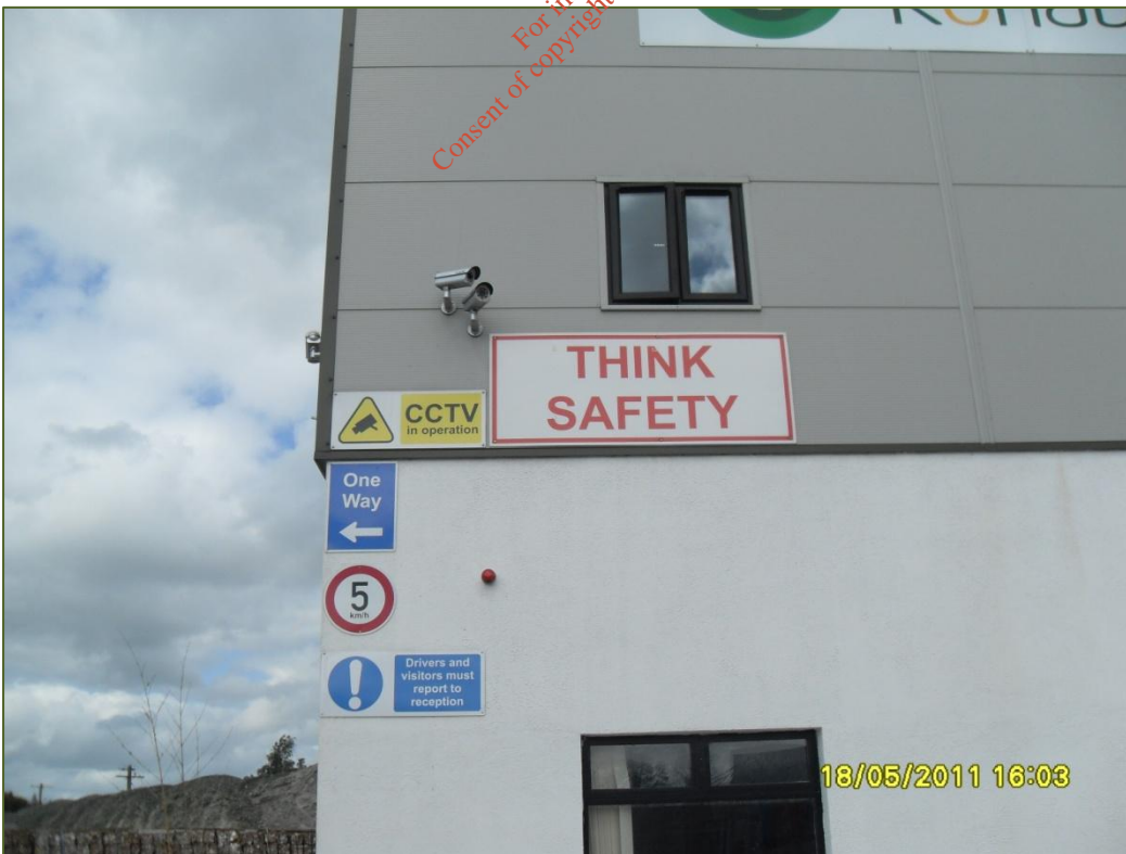
Photograph D.1.2: CCTV camera positions on Main Process Building
