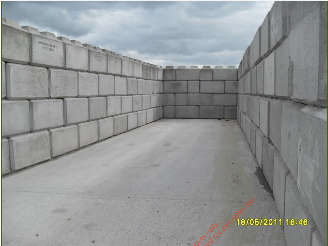
Photograph D.1.11: Storage bay
