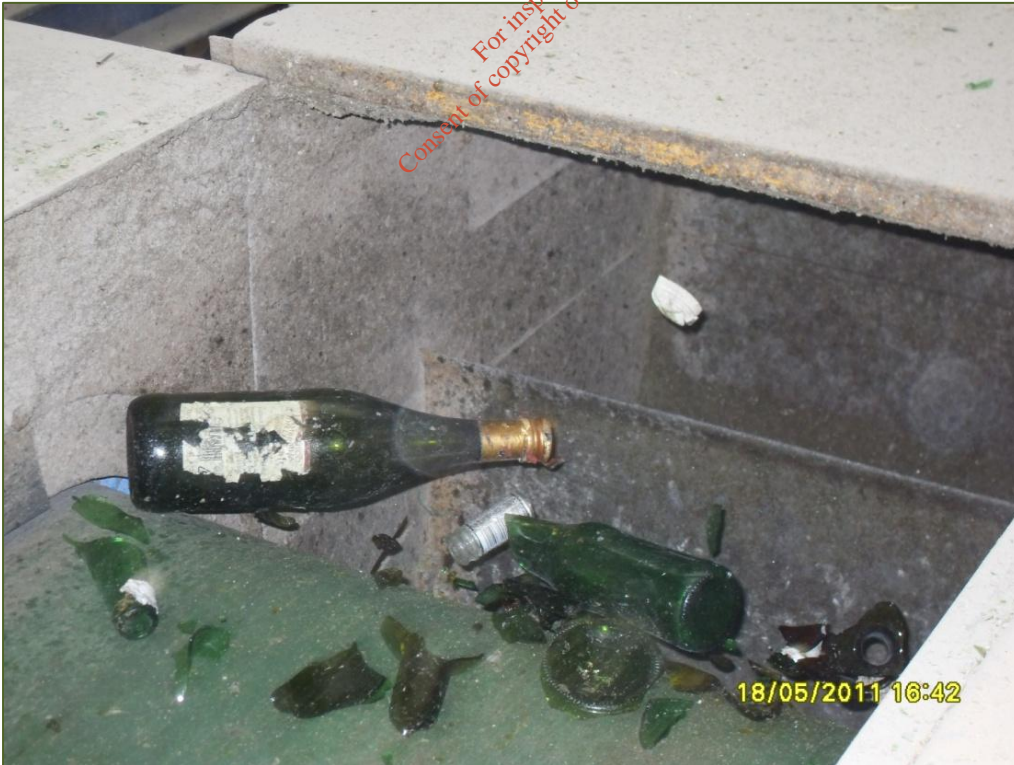
Photograph H.3.1: Eddy Current Separator Unit
