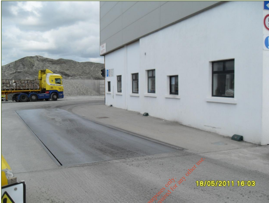
Photograph D.1.7: Weighbridge position and operator's window
