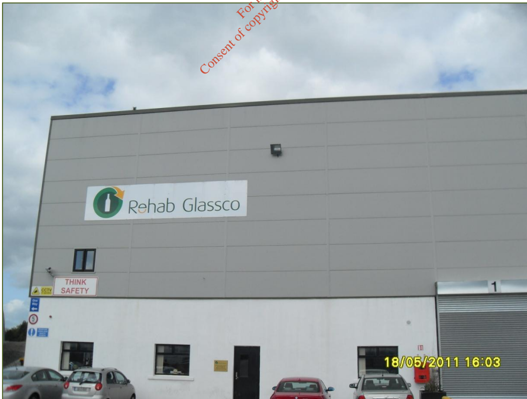
Photograph D.1.14: Site offices located at western side of Main Process Building
