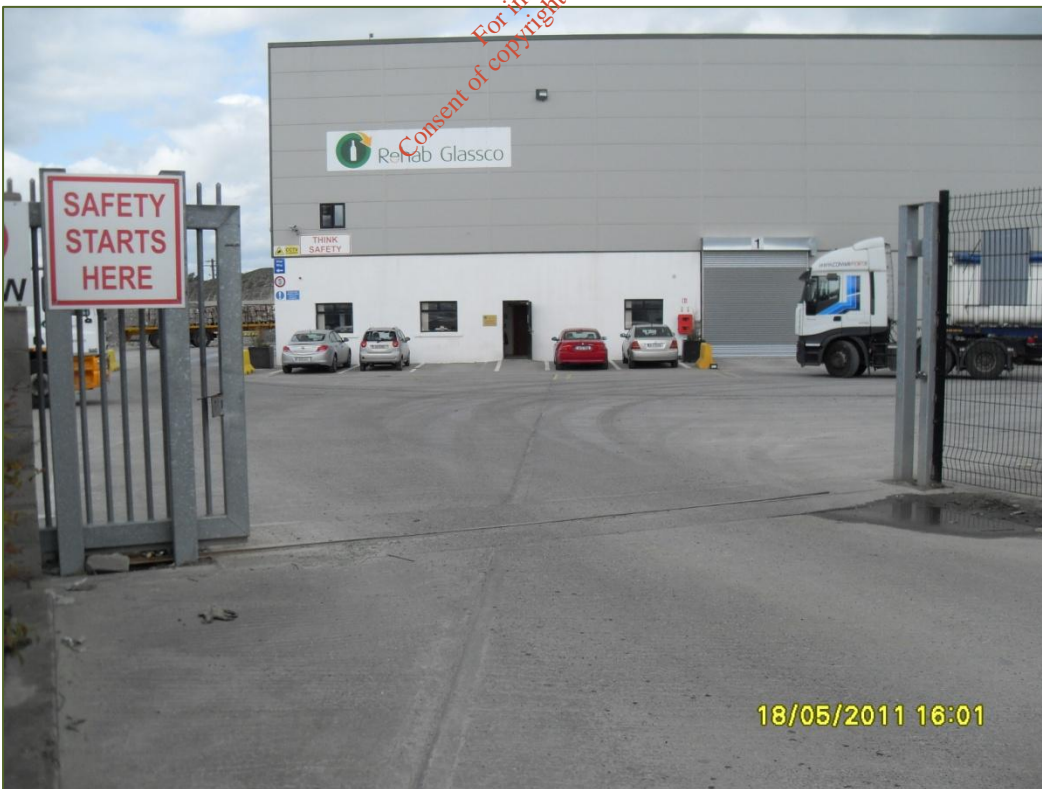
Photograph D.1.4: Site roads – concrete hardstanding
