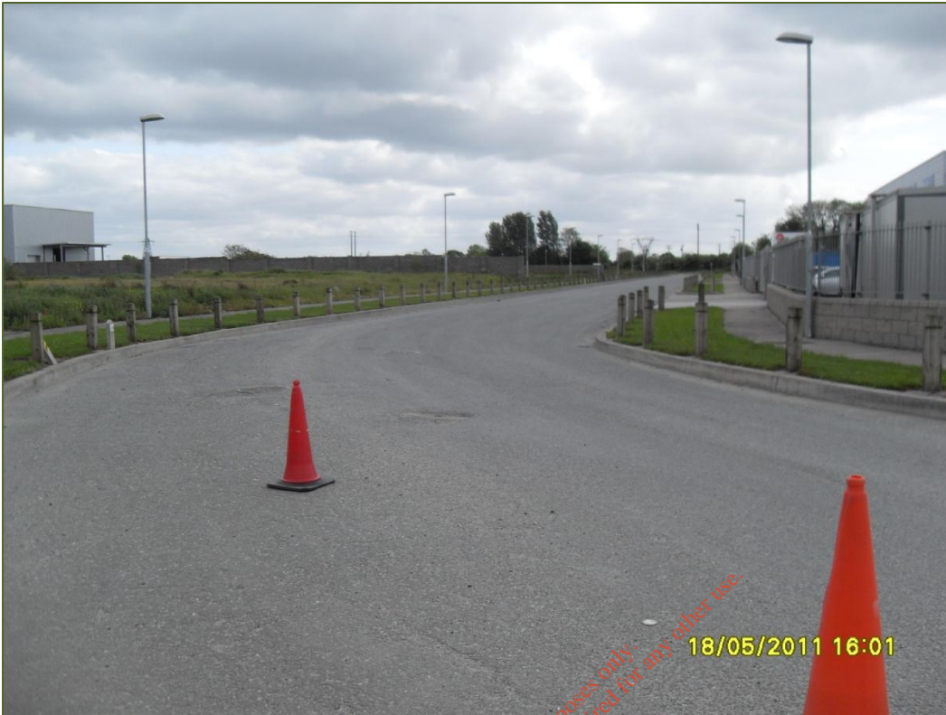
Photograph D.1.3: Access Road, Osberstown Industrial Park
