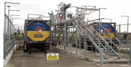
Figure 1.2.4 Picture of Tanker Loading/Unloading Bay
