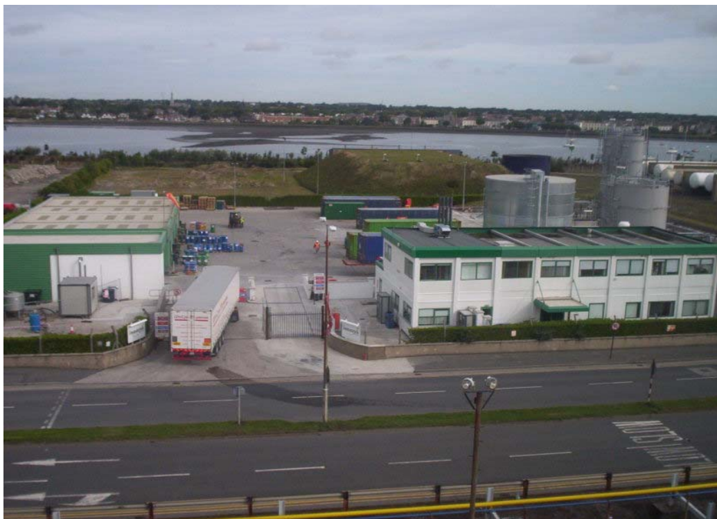
Figure 1.2.1 Picture of Dublin Port HazWaste Facility
