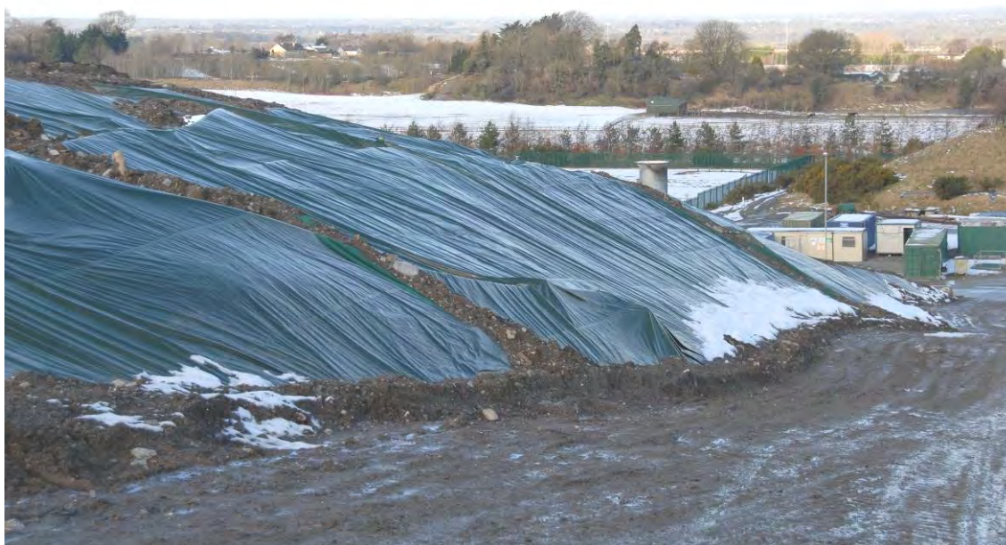
Plate 5: CoverTop 32 placed on side slopes of Cell 14. (Enclosed Flare in background)
