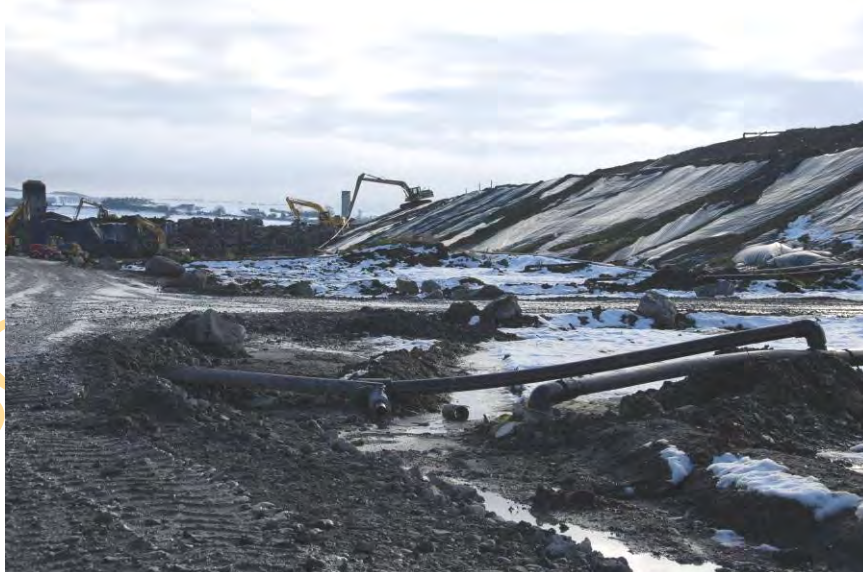
Plate 4: CoverTop 32 placed on side slopes of Cell 14.
