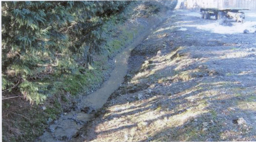
Surface water ditch, Southern boundary, 14 th December 2010.
