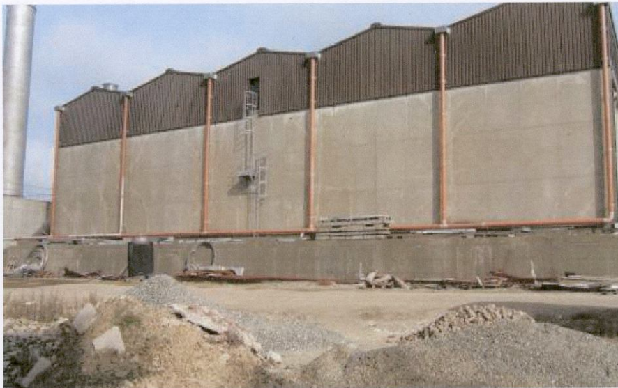
Appendix 3. New roof water collection system, taken 1 st September 2010
