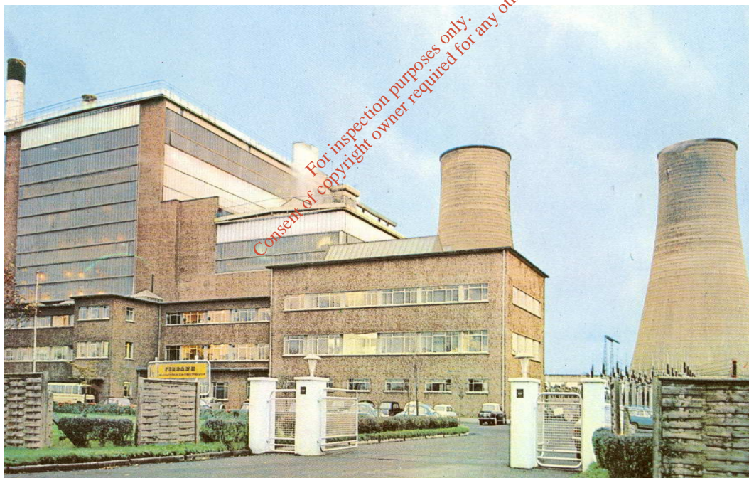
Figure 2.2 View from Entrance to the Former Ferbane Peat Fired Station
