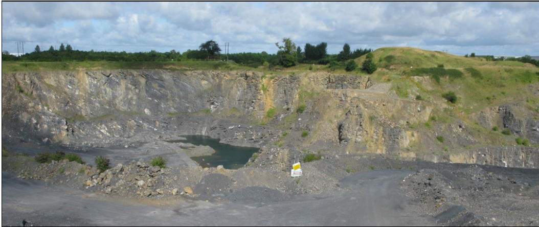
Plate 5-1 Limestones Exposed in Western Face of the North Quarry. Note steep dip to north-west and well-bedded nature of the limestones.
