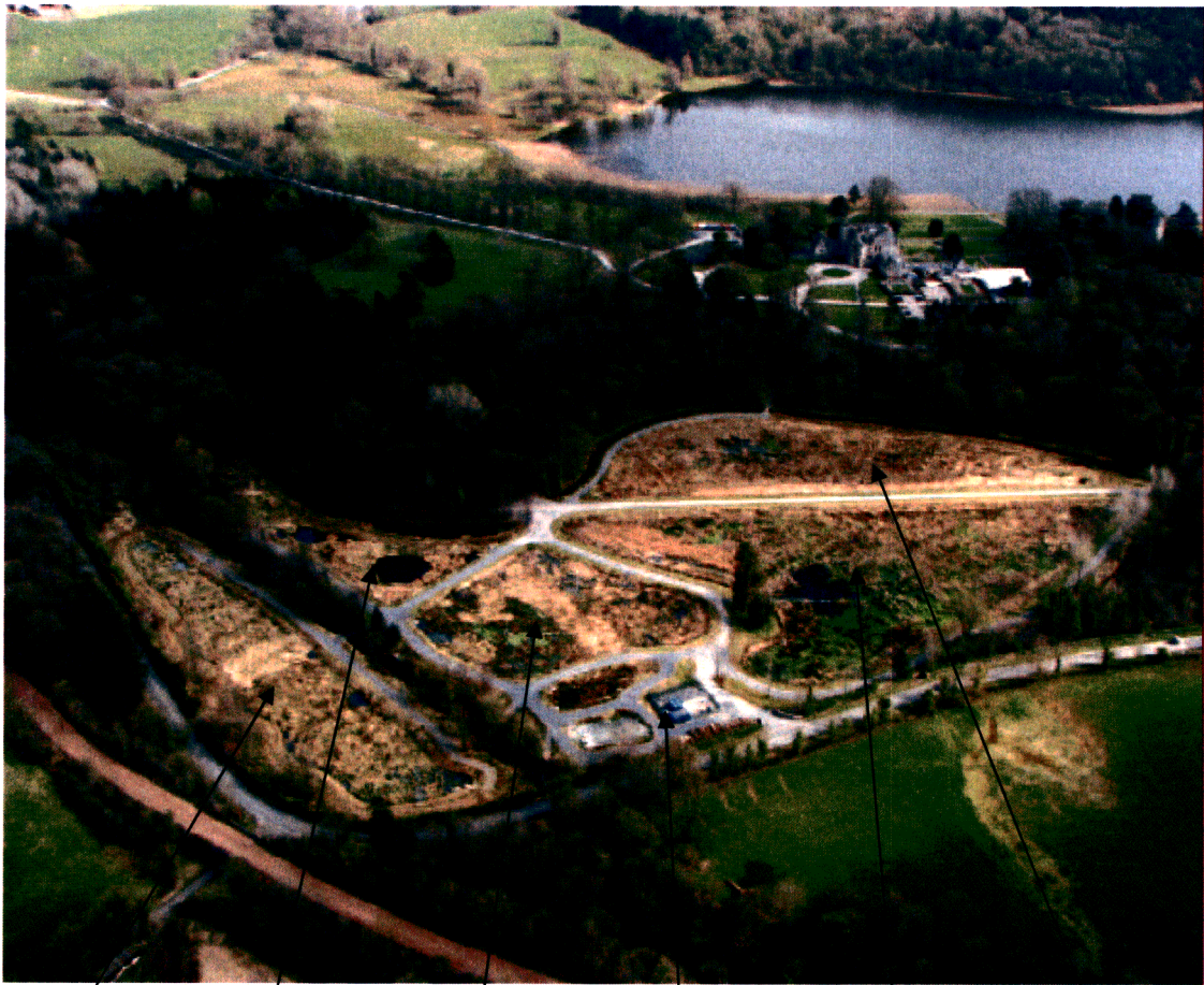
Figure 3.0 Glaslough Integrated Constructed Wetland
