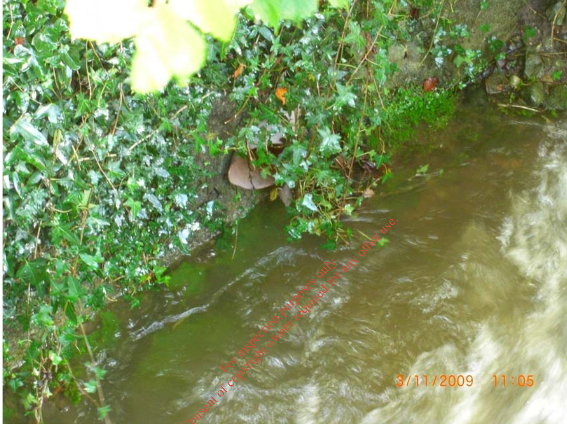
Photo – KK-WWDL-213-C.1.2.1 – Storm Water Overflow at The Siphon at Quinn's Garage
