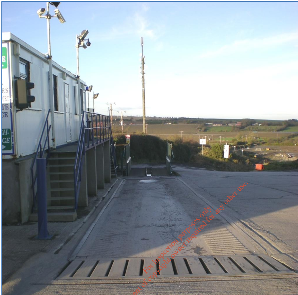
Photograph D.5: Weighbridge (existing infrastructure)
