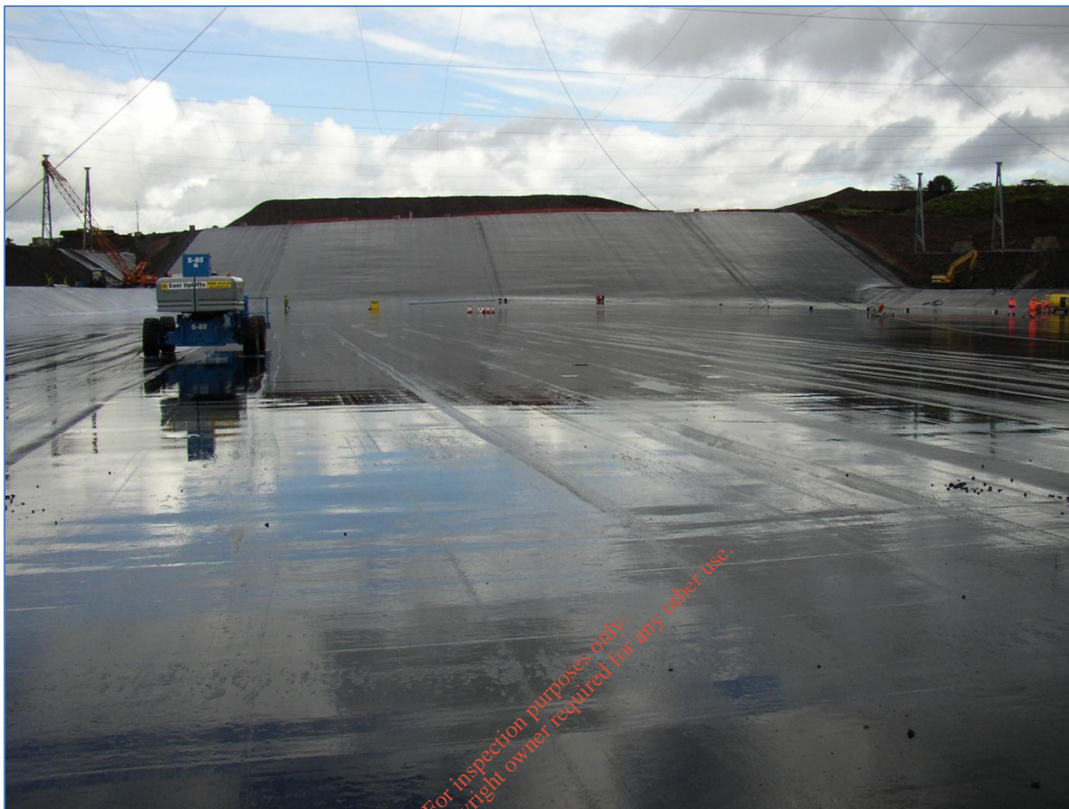
Photograph D.23: DAC liner photograph#3
