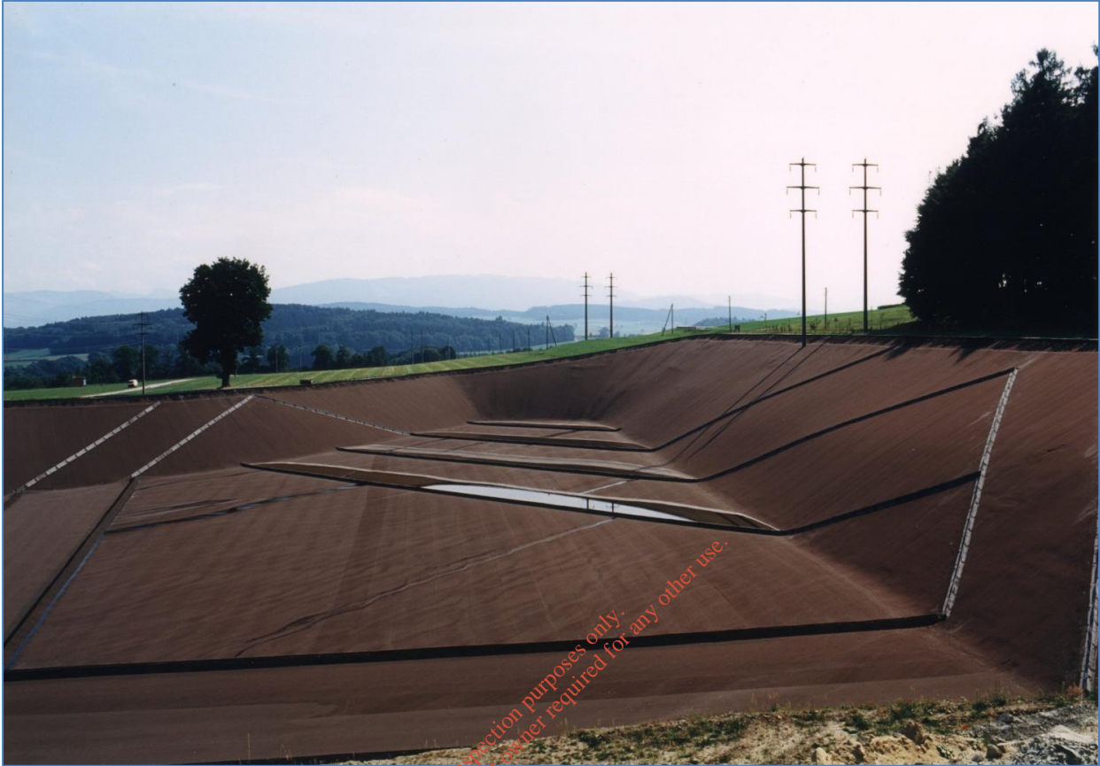
Photograph D.32: Rainwater deflectors commonly used on DAC-lined cells
