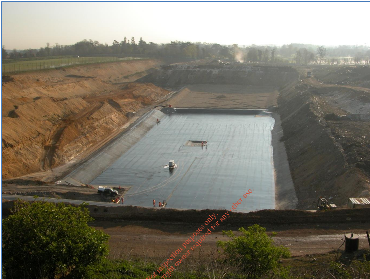
Photograph D.22: DAC liner photograph#2
