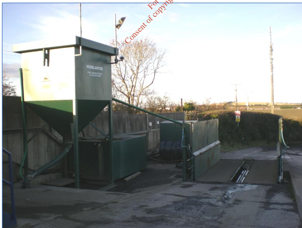
Photograph D.7: Wheelwash (existing infrastructure)
