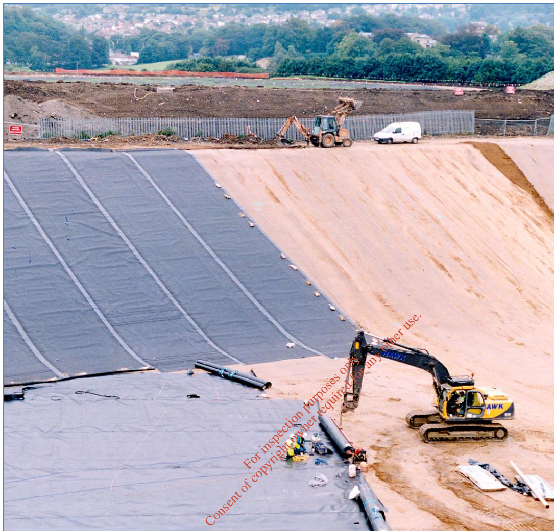
Construction of High-density Polyethylene (HDPE) Liner Landfill Site, UK
