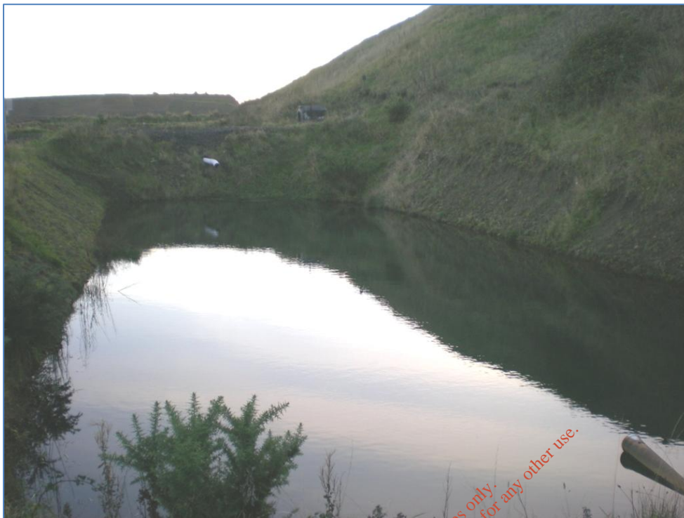
Photograph D.14: Settlement Ponds (existing infrastructure)
