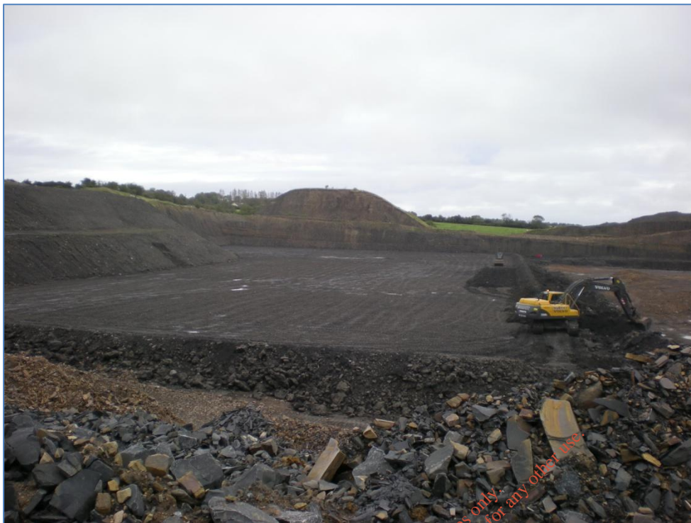
Photograph D.18: Inert Cell 4 (existing infrastructure)
