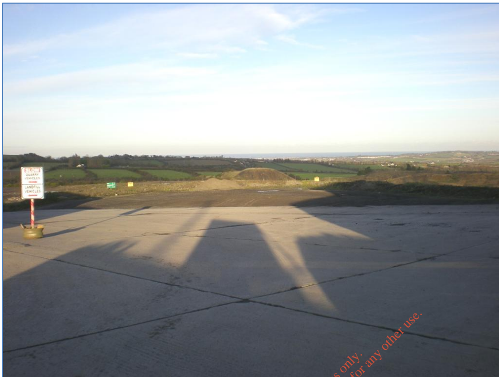
Photograph D.4: Garage and Car Park Hardstandings (existing infrastructure)
