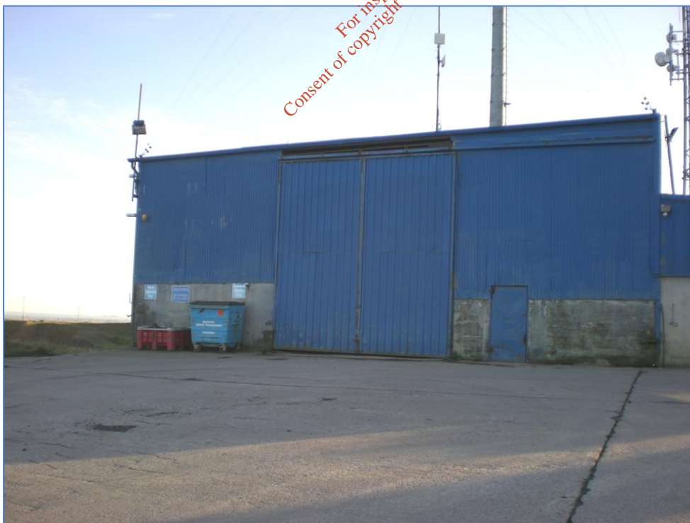
Photograph D.15: Maintenance Building (existing infrastructure)
