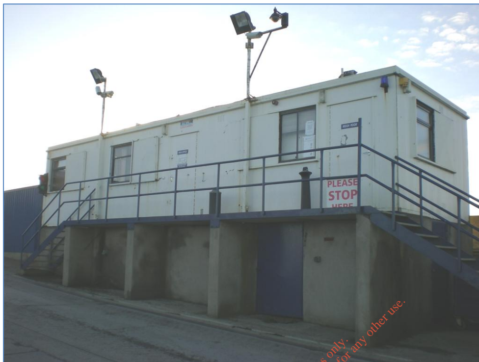
Photograph D.16: Site Office (existing infrastructure)
