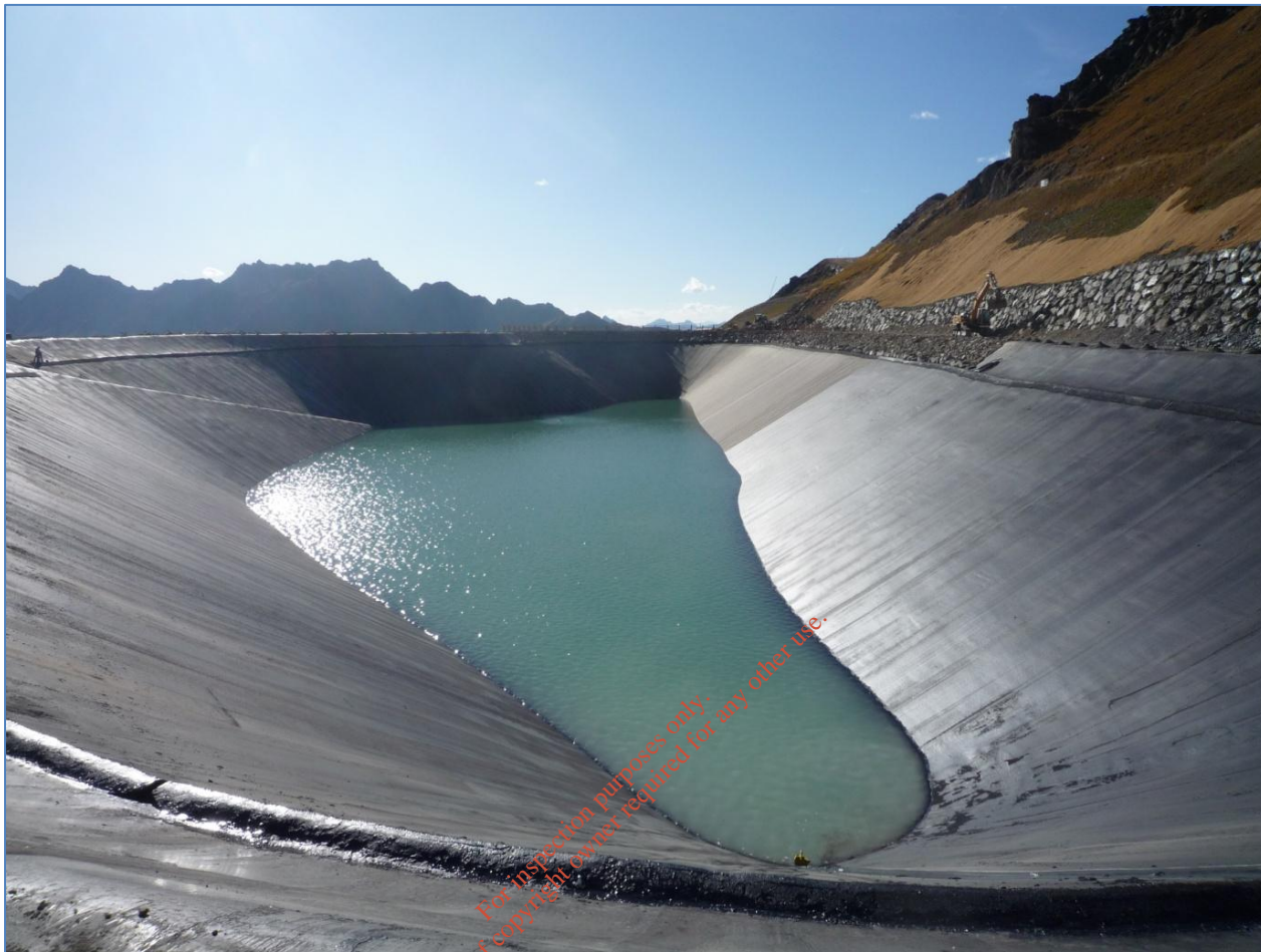
Photograph D.21: DAC liner photograph#1
