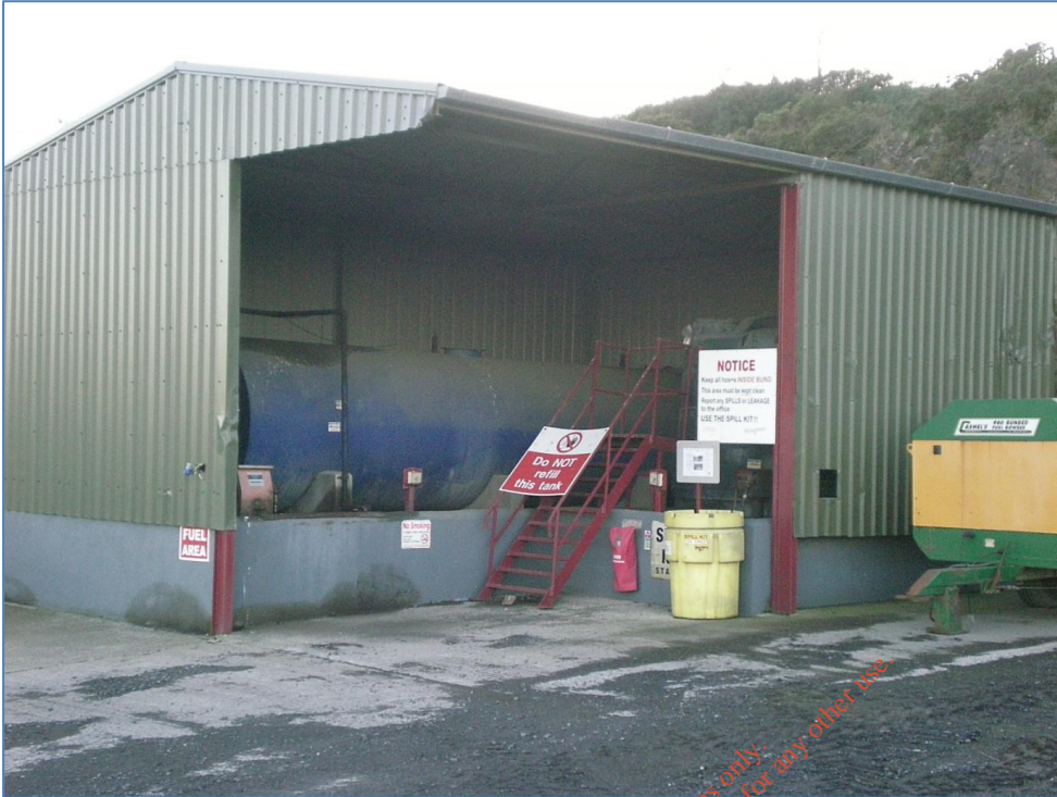
Photograph D.10: Bunded and roofed fuel storage area (existing infrastructure)
