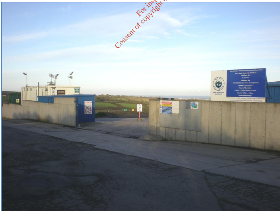
Photograph D.1: Existing Facility Entrance (existing infrastructure)
