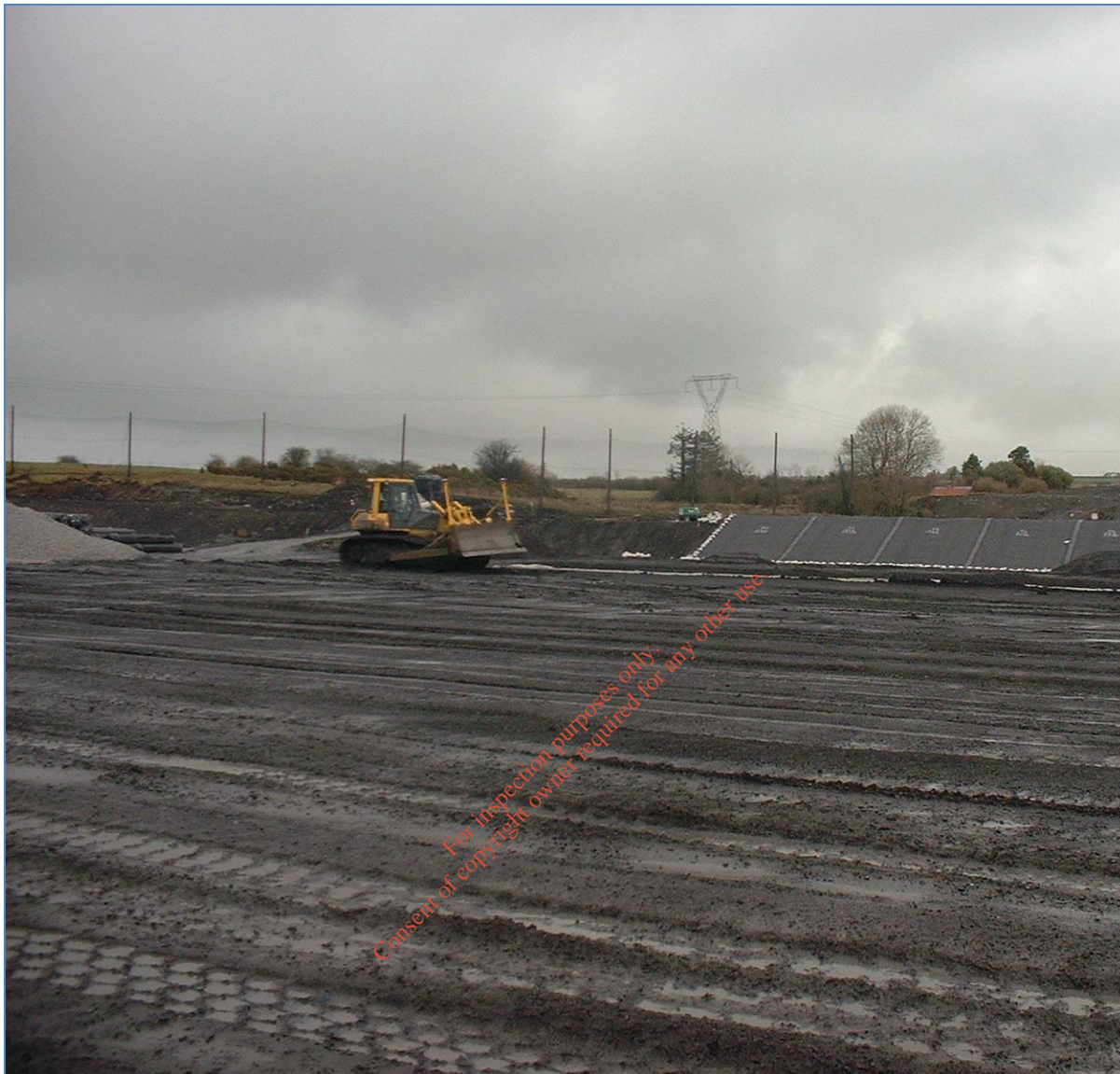
Construction of Waste Cell to Formation Level
