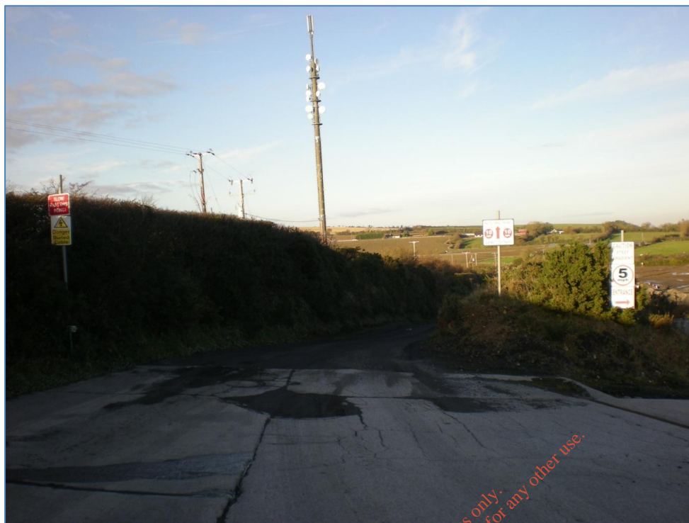
Photograph D.12: Traffic Control Signage (existing infrastructure)
