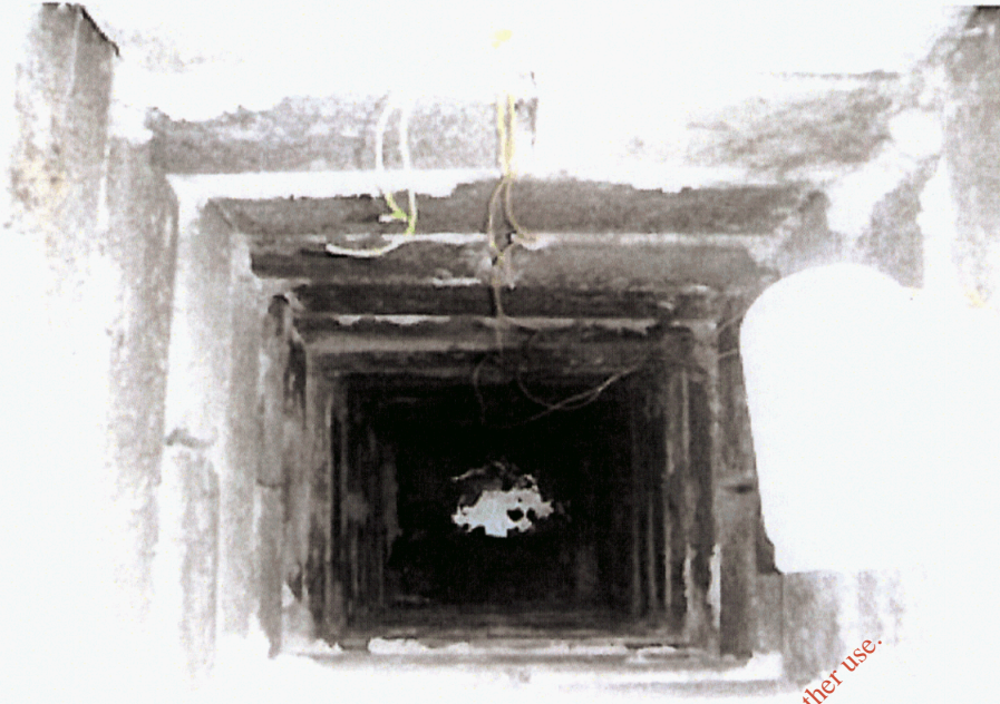
Photograph 3: Storm water monitoring point SW2, with internal dipper.
